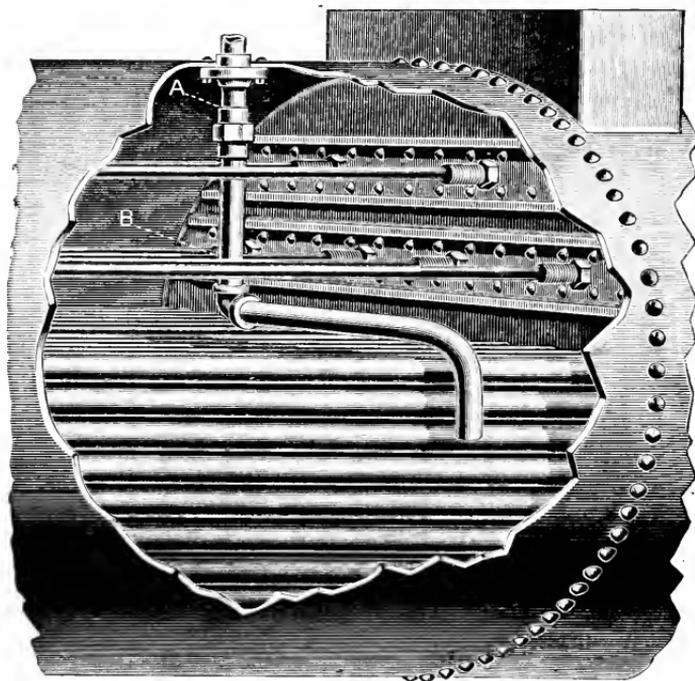
FIG. 1. — ARRANGEMENT OF THE FEED PIPE AND BRACES.
