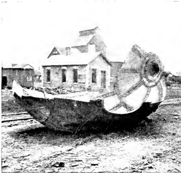
FIG. 2.—AN EXPLODED ROTARY.
