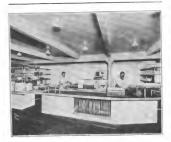
CHINA WASHING DEPARTMENT, (Davenport-Hotel, Spokane): Blakesiee No. 80 Niagara motor driven machine. Van's new style metal dish tables. Baskets filled and sild to feed end of the machine, passing thru it from right to left and landing on the clean dish assorting table. Tray rack under dish table. Trays are washed in sink in front of the machine (see faucets over tray). Note sanitary enclosure of the dish table.
