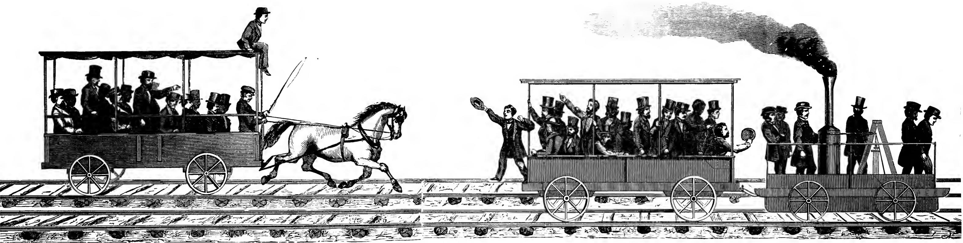
The trial took place on the Baltimore and Ohio Rail-Road, on the 28th August, 1830. The sketch represents the moment the Engine overtook and passed the Horse-Car, the passengers filled with excitement.
