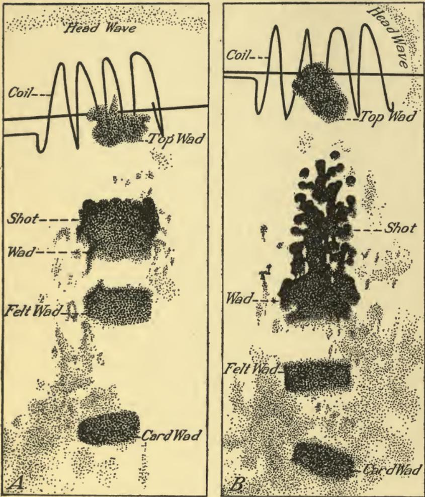
FIG. 80.—Photographs of shotgun charges leaving the muzzle, the camera being snapped by contact of the forward wad against the wire. *A* shows the shot leaving an ordinary barrel in a compact body, while *B* reveals the shot from the choke-bored barrel stringing out for the reasons explained in the text.
