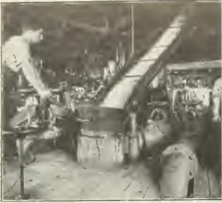
Beet pulp and juice flowing into tanks for diffusion with water
