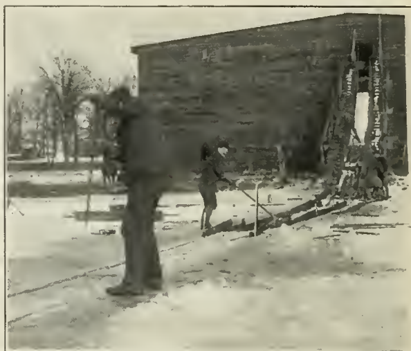
Filling the local ice-house
