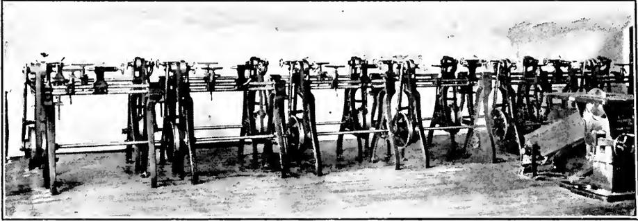
Fig. 32. Wood Turning Equipment Without Overhead Shafting.
