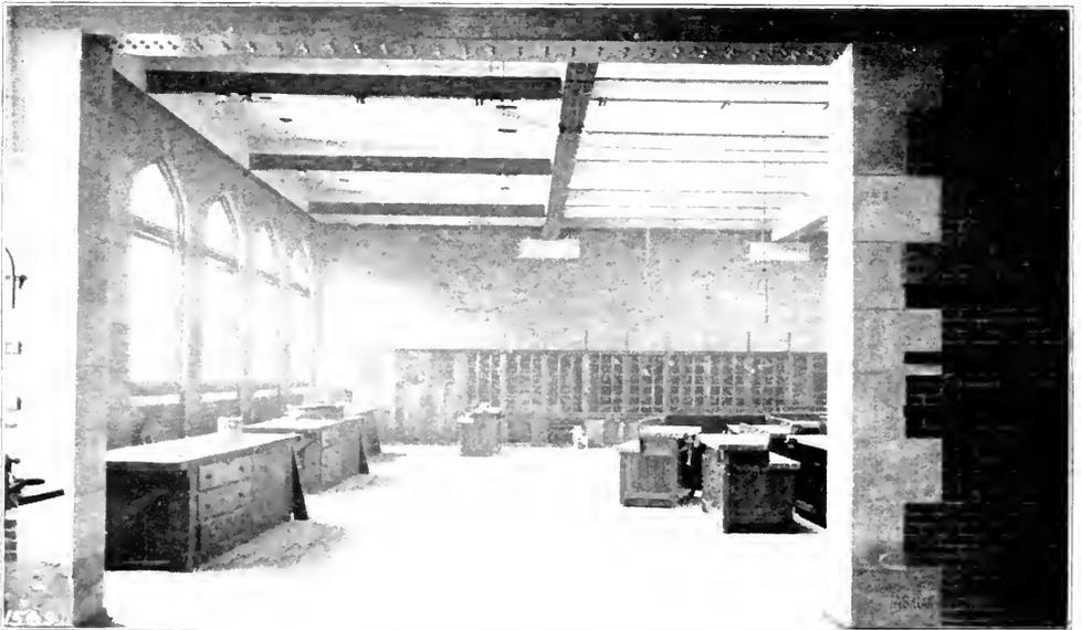
Fig. 67. Pattern Shop Chicago Manual Training School, showing Distribution of Light from Saw-Tooth Roof.
