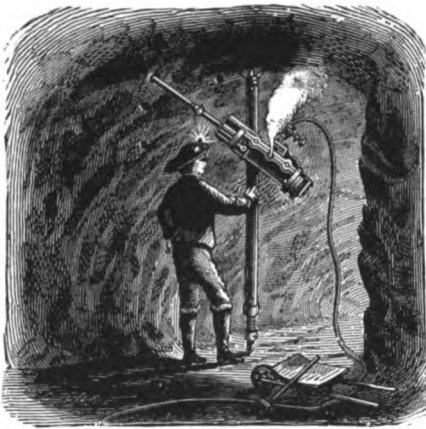
Fig. 629.—THE INGERSOLL ROCK-DRILL IN WORK.
