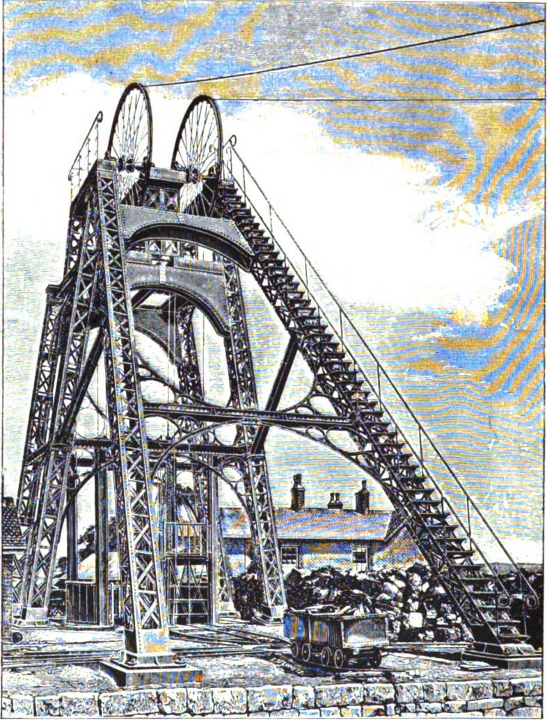
Fig. 67.—PIT-HEAD FRAME ERECTED BY MESSRS. THORNEWILL & WARRHAM AT THE NEW HALL PARK COLLIERIES.
