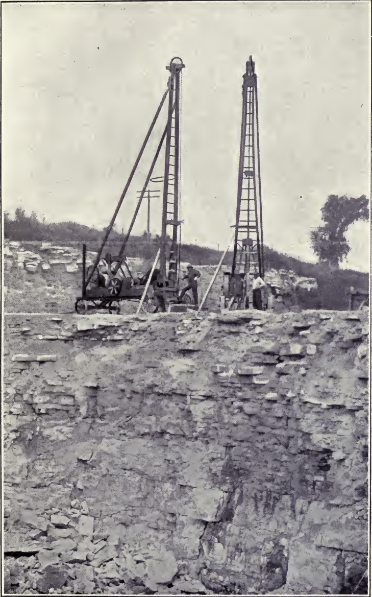
BIG BLAST HOLE DRILLS IN OPERATION.
