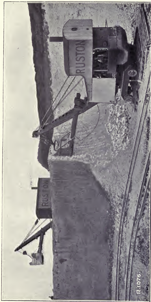
Showing the usefulness of the CRANE NAVVY in quarry work. The machine at the top is removing the top soil or overburden, and the machine in the bottom is excavating the mineral, which in this case is chalk for making cement.
