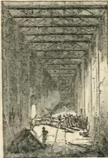
PLATE GLASS CASTING. BRINGING OUT THE POT.
