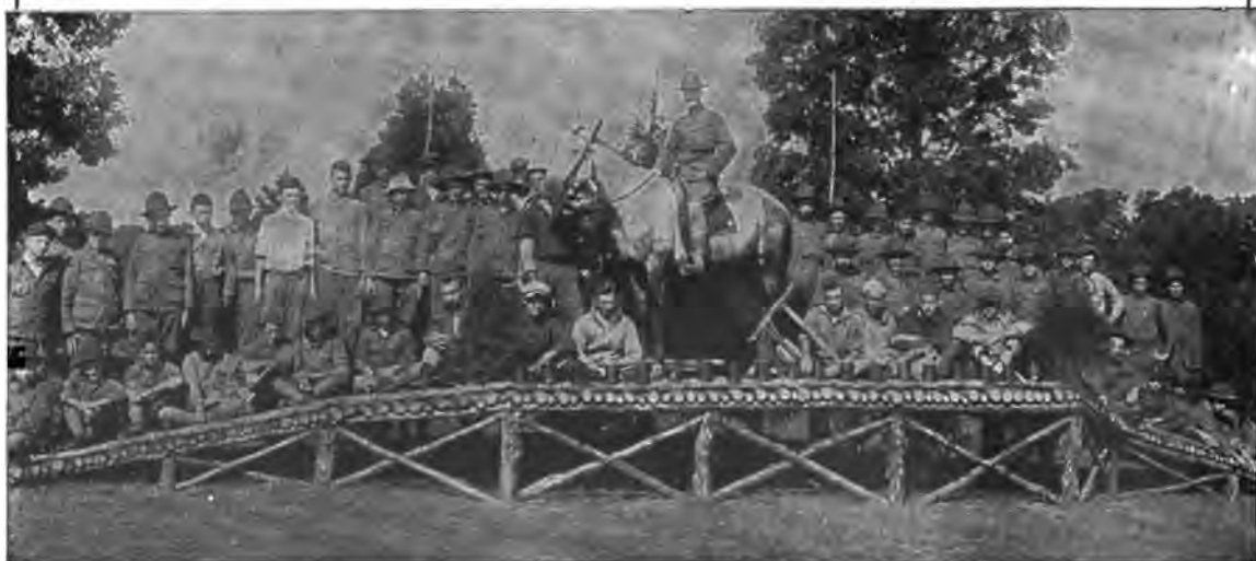
Rustic Bridge constructed by St. Louis scouts. One of the tests for the Pioneering Merit Badge
