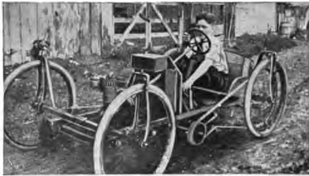
Donald Mitchell, Topeka, Kan., Put This Automobile Together—Bicycle Wheels in Front, Motorcycle Wheels Behind; Rubber Be't from Motor to Rear Wheel.
