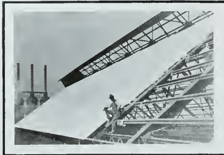
ASBESTOS CORRUGATED ROOFING BEING APPLIED
