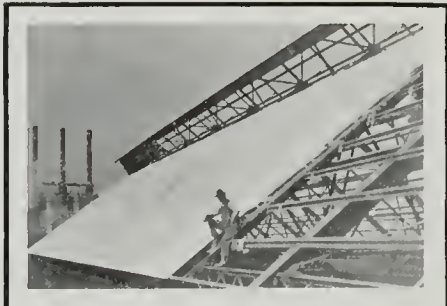
ASBESTOS CORRUGATED ROOFING BEING APPLIED
