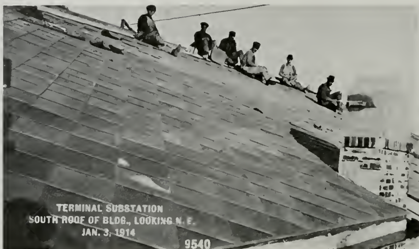
APPLYING "AMBLER ASBESTOS SHINGLES" TO ROOF
