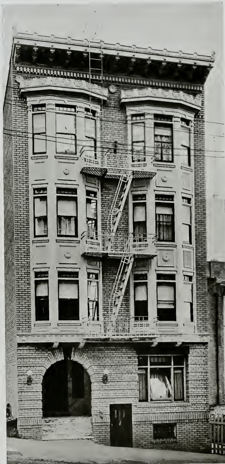
RULFS APARTMENTS, SAN FRANCISCO ROUSSEAU & ROUSSEAU, ARCHITECTS
