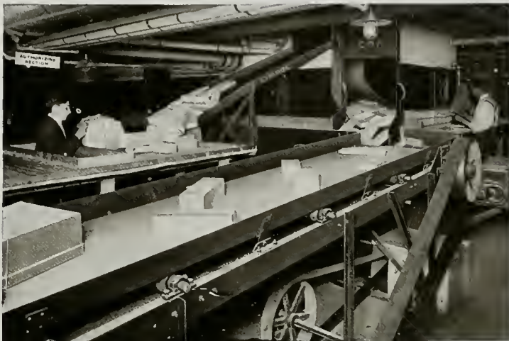
Belt Conveyors receiving packages from outlets.
