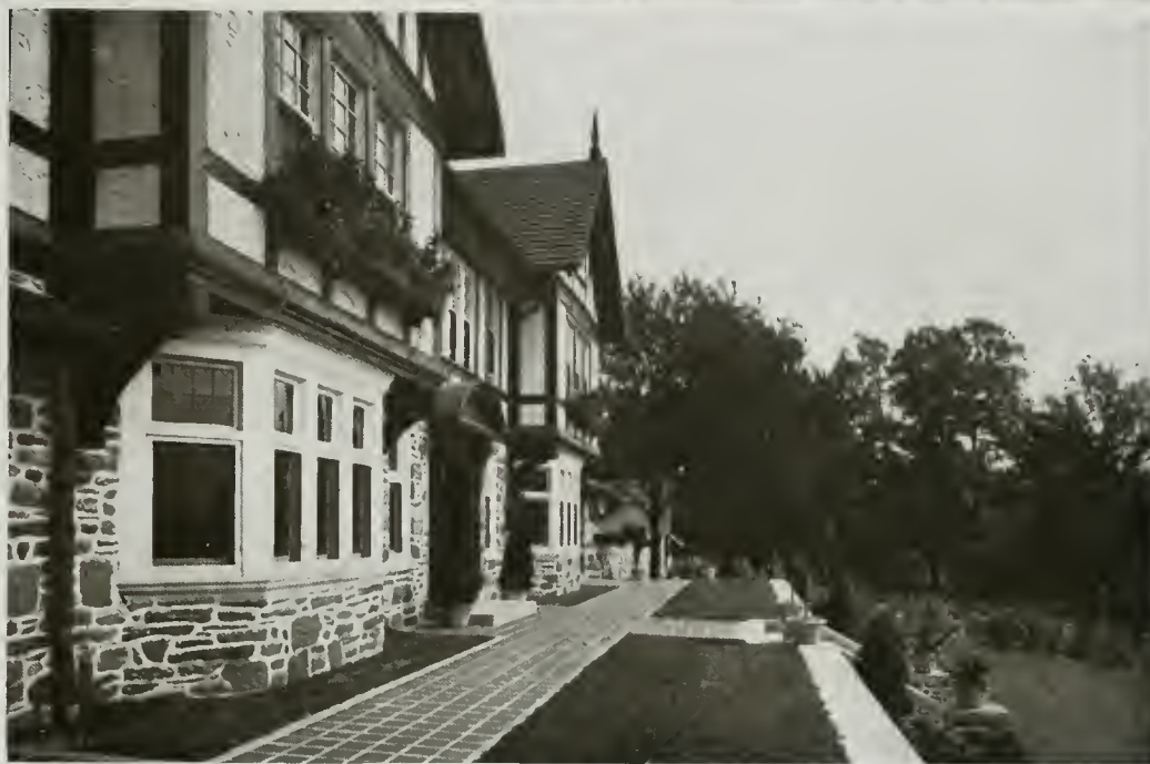
Atlas-White used for pointing, setting and for stucco
