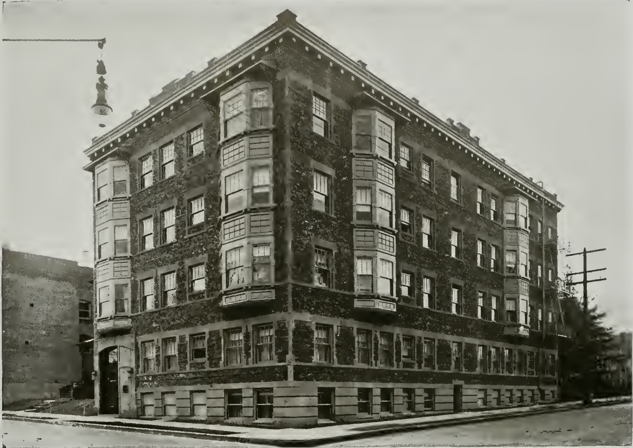
BRETNOR APARTMENTS, PORTLAND CLAUSSEN & CLAUSSEN, ARCHITECTS
