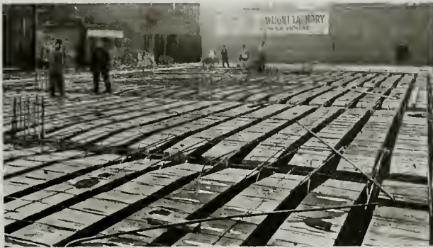
STEELFORMS READY FOR CONCRETE
