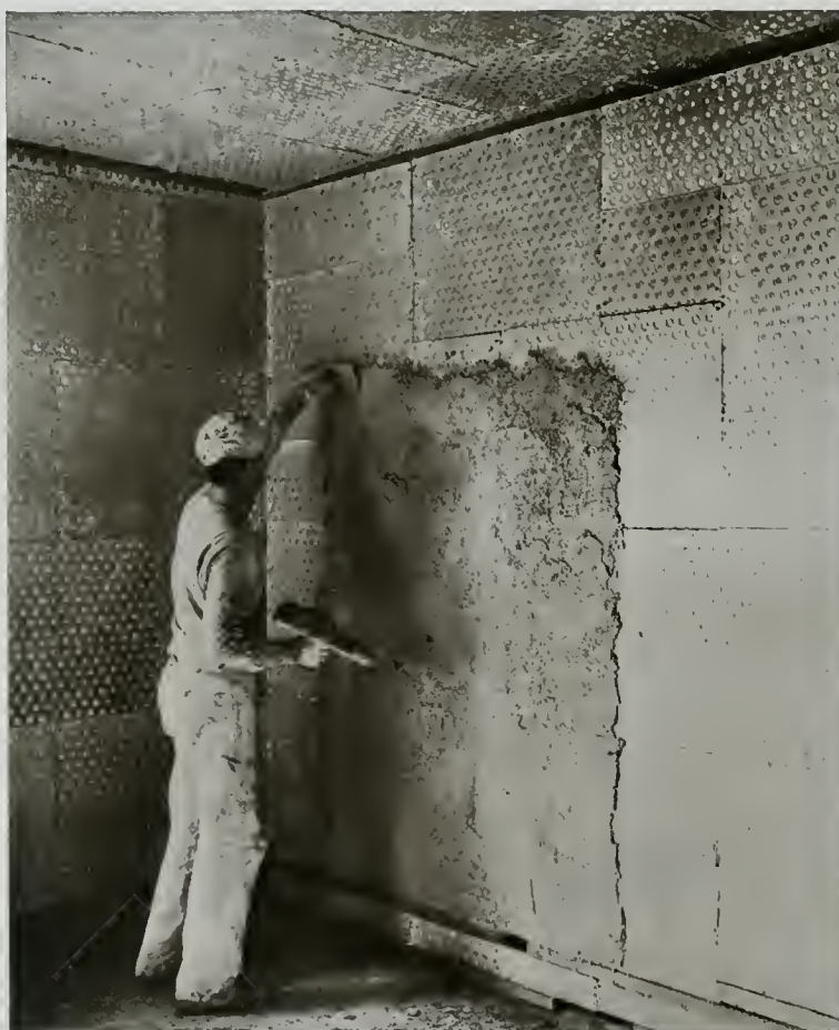
A BUTTONLATHED ROOM IN THE MAKING
