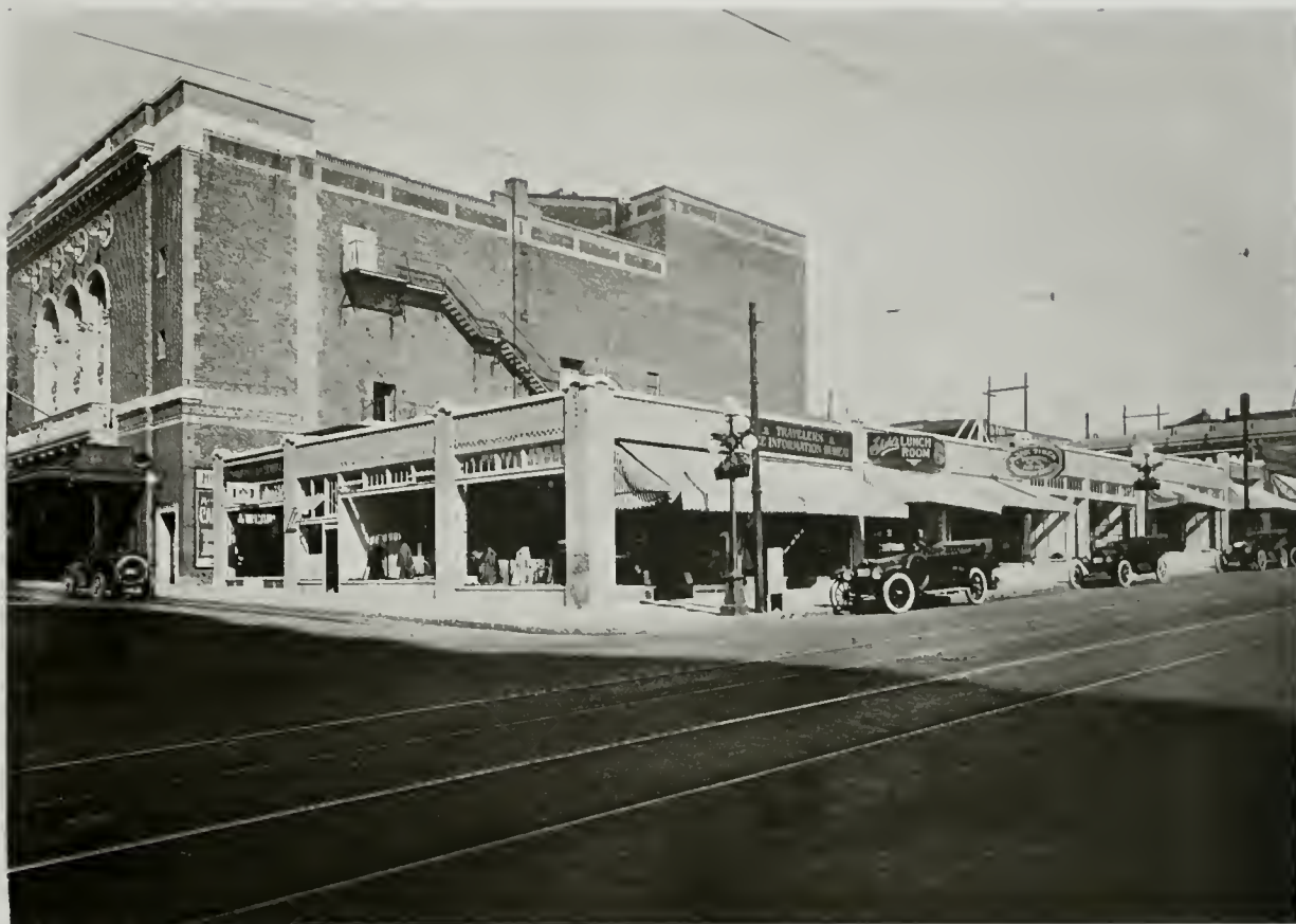
NEYHART BUILDING AND METROPOLITAN THEATRE, SEATTLE
