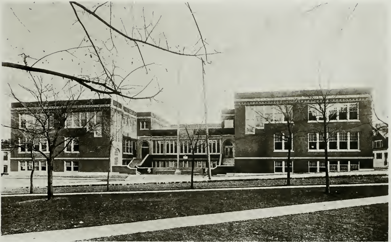
GENERAL VIEW OF ENTRANCE FRONT
