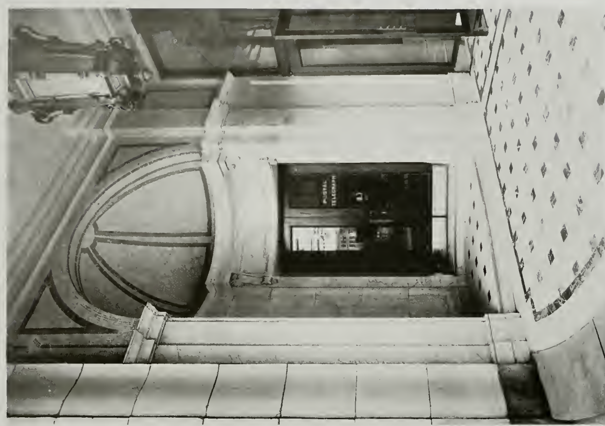
VESTIBULE OF WHITE BUILDING, SEATTLE
