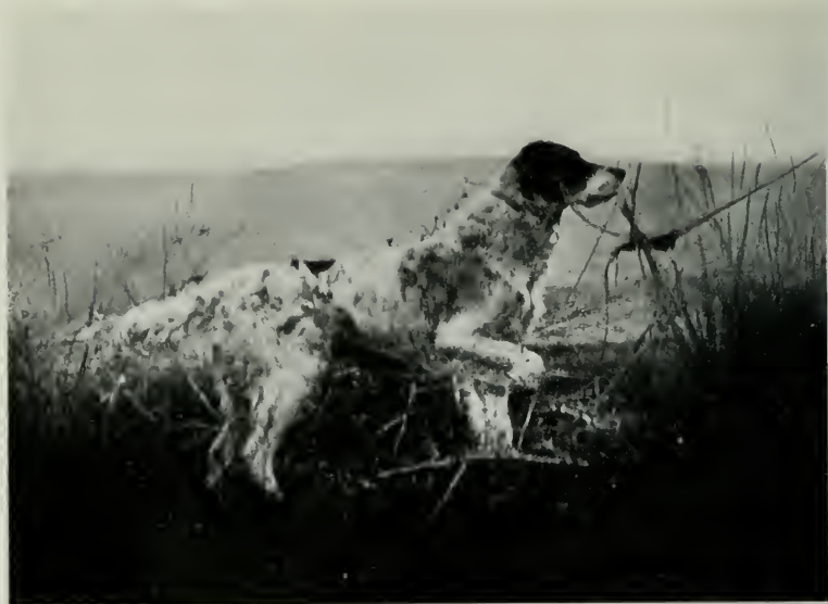
MOMONEY II, A CRACK FIELD TRIAL SETTER
