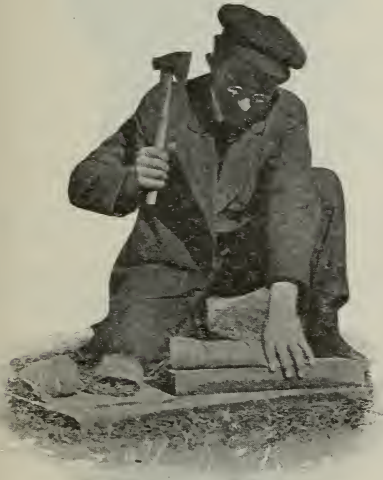
Chopping up rolls of burlap for smoker-fuel. An old sack is rolled up, tied at intervals, and then cut in pieces between the strings.
