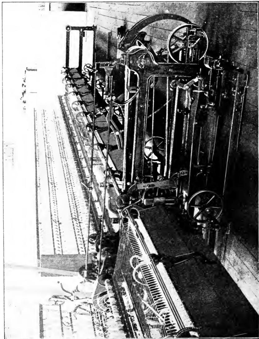
Always used for wool. **MULE DRAWING AND SPINNING FRAME]** Part of the machine moves away from the frame, thus drawing out the thread, which is then twisted.
