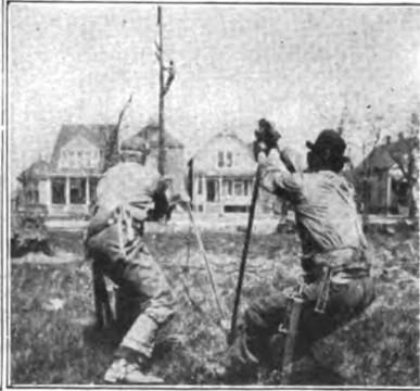
Fig. 11.—View Showing Method of Straightening Pole.
