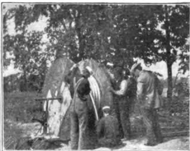
Fig. 23.—Feeding Cable Into Vault.
