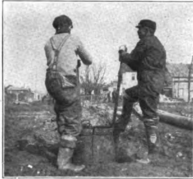
Fig. 12.—View Showing Method of Using Iron Barrel in Digging Pole Holes In Soft Ground.
