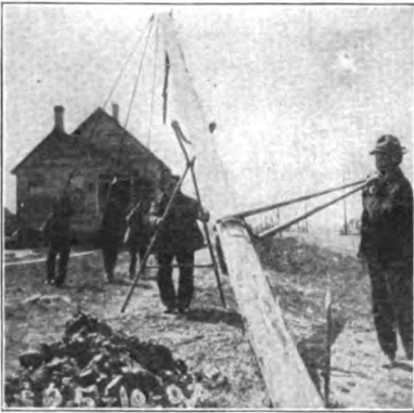
Fig. 10.—View Showing Method of Raising Pole.
