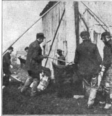
Fig. 13.—Removing Iron Barrel with Bars.
