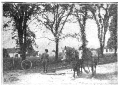
Fig. 24.—Pulling Cable.
