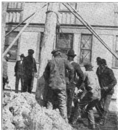
Fig. 14.—Removing Iron Barrel with Block and Tackle.
