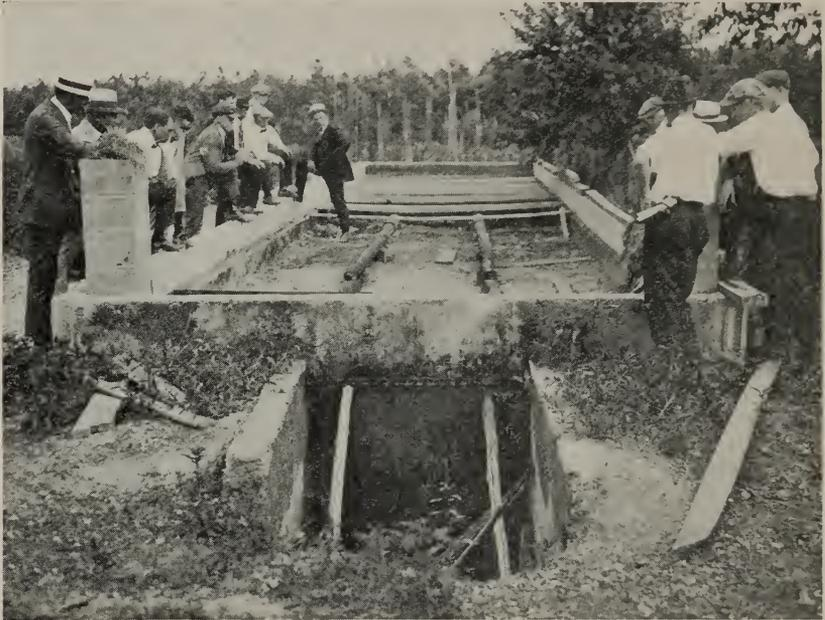
Fig. 4.—Top view of fire-heated hotbed, concrete construction. (Courtesy New Jersey Experiment Station.)
