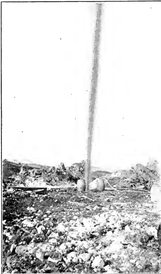
FIG. 32.—Drill-hole being sprung.
