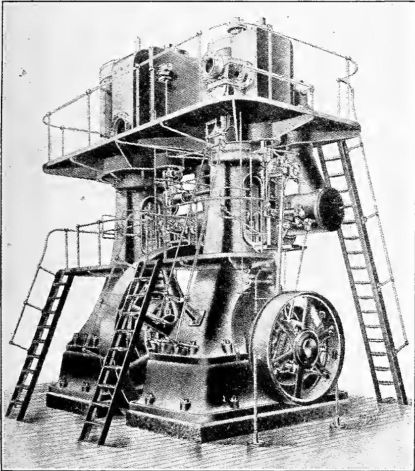
Fig. 25. Buckeye Vertical Cross-Compound Engine
