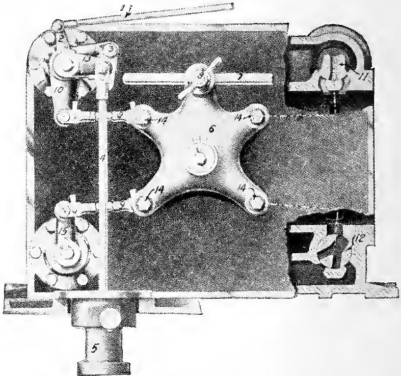
Fig. 27. Corliss Valve Mechanism in Detail
