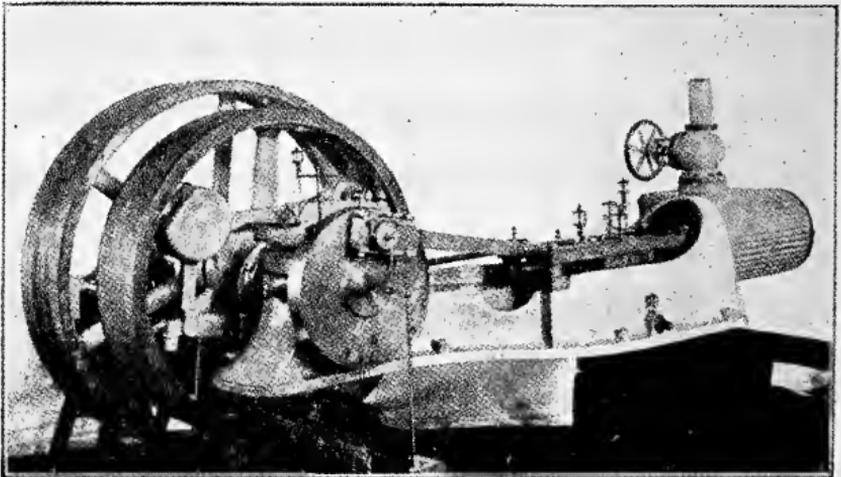
Fig. 23. Simple Slide Valve Engine of Side-Crank Type
