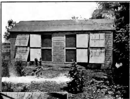
Fig. 3.—Aurora Leghorn Farm's "Style B" house, a modified glass front house. Note the wire screen doors with muslin frames hooked back for summer use and the windows open.
