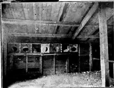
Fig. 2.—Interior of "Style A" house showing clear floor space, droppings board, method of bolting sections together and of fixing roof timbers. A, exterior and interior view of trapnest; B, exterior and interior view of trap sprung by hen on entering, C, trap unset and shoved out of the way.
