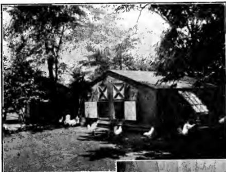
Fig. 1.—Aurora Leghorn Farm's portable modified Tolman Fresh Air House, "Style A," size 14x14. Note muslin screens. The house is raised off the ground, allowing free circulation of air, thus preventing dampness.
