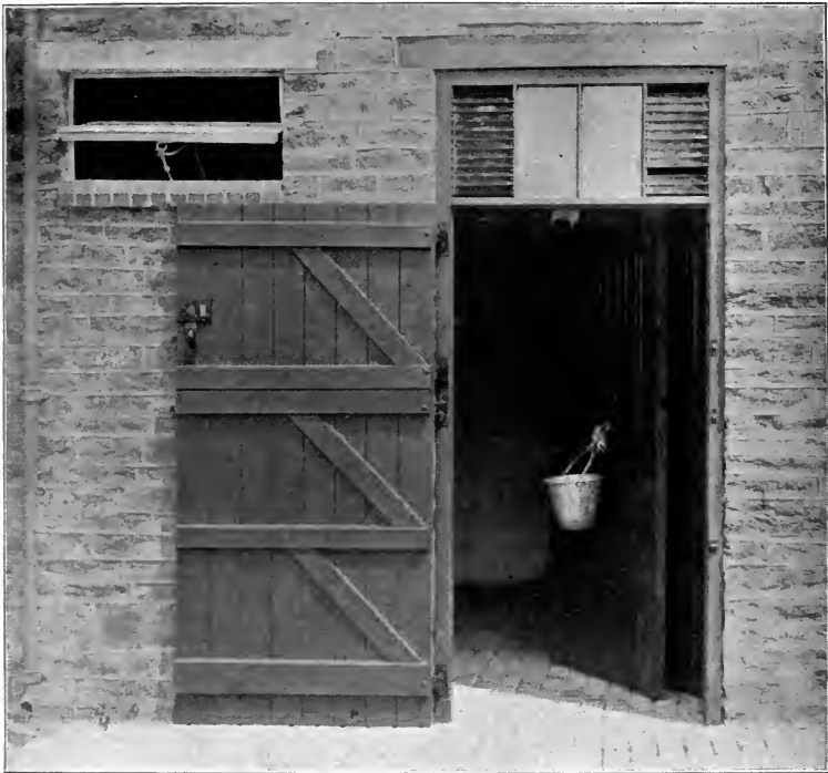
Fig. 27. Water bucket fixed to door of box.
