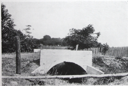
Figure 20. Arch Bridge, Marion County, Indiana. 8-foot span; 2-foot rise; 18-foot roadway. Cost $550.
