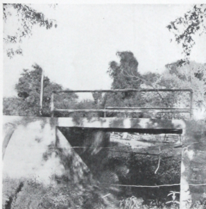
Figure 4. Concrete Bridge, McLean County, Illinois. 12-foot span; 16-foot roadway; Cost $300.
