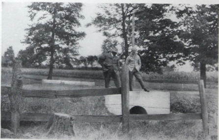
Figure 48. Concrete Culvert, McLean County, Illinois. 42-inch diameter; 20 feet in length. Built by Township Commissioners in 10 hours over Merrillat culvert forms. Cost, exclusive of form, $62.50.
