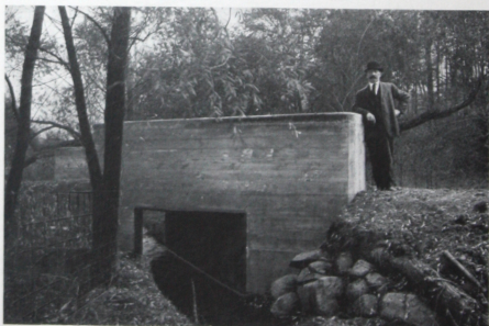
Figure 12. Concrete Culvert, Town of West Bloomfield, Ontario County, New York. Designed by New York Highway Commission. Span 4 ft. Roadway 22 ft. Cost $375. Culvert has been built at an angle to the axis of the stream flow.
