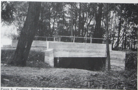
Figure 9. Concrete Bridge, Town of Gorham, Ontario County, New York. Designed by New York Highway Commission. Span 18 ft. 6 in., Roadway 23 ft. Built by town labor. Cost $188.
