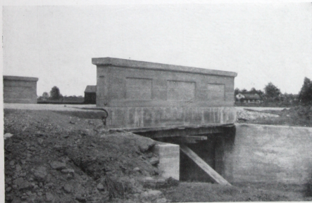
Figure 8. Flat Slab Bridge, Wayne County, Michigan. 9-inch slab; 12-foot span; 18-foot roadway, reinforced with 1-inch twisted bars, on 11-inch centers. Cost $400.
