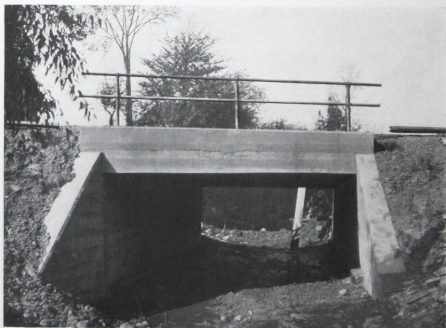
Figure 10 Concrete Bridge, Town of Canandaigua, Ontario County, New York. Designed by New York Highway Commission. Span 14 ft., Roadway 26 ft. Built by contract. Cost $950.
