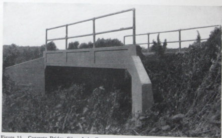
Figure 15. Concrete Bridge, Silver Lake Township, Martin Co., Minnesota. 20 foot span. 18-foot roadway Cost $734.
