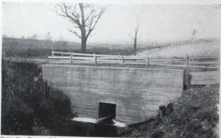
Figure 22. Concrete Culvert, Milo, Yates County, New York. Designed by New York Highway Commission. Culvert Head Walls 40 feet long, 16 feet high; opening 5 feet x 6 feet. Built with town labor at a cost of $636.
