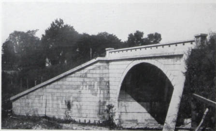
Figure 18. Concrete Arch Bridge, Marion County, Indiana. 20-foot span; cost $1,500. This bridge is of monolithic concrete construction but marked in imitation of stone masonry.
