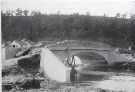
Figure 47. Luten type reinforced concrete bridge near Holliday's Cove, West Virginia, which withstood unusual flood conditions, the only damage being to the concrete railing which was shattered by the debris carried by the flood.
