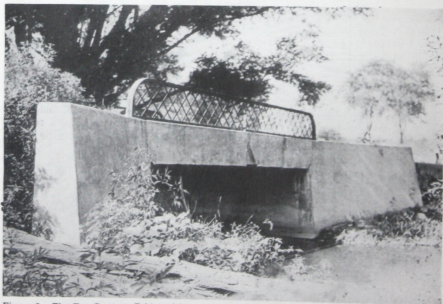
Figure 6. Flat Top Concrete Bridge with ornamental iron guard rail, near Geneva, Illinois.
