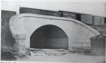
Figure 50. Concrete arch bridge on the P. C. C. & St. L. Railroad, Columbus, Ohio, built in 1909. The flood at this point was of such a character that the brick pavement underneath the bridge was entirely washed away leaving only the concrete foundations.
