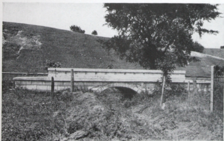
Figure 30. Concrete Arch Culvert, Marion Co., Indiana. 6-foot span; 3 1/4-foot rise; 18-foot roadway. Cost $700. This bridge is of monolithic construction marked in block form.
