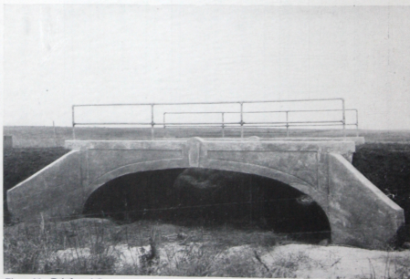
Figure 26. Reinforced Concrete Arch Bridge, Iroquois, South Dakota, 20-foot Span, 18-foot roadway. Designed by Missouri Valley Engineering Company, R. S. Warner, Contractor.
