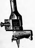
Irwin Bit.—The Irwin bit is sometimes called the solid center bit. It is a fast borer, having a coarse pitch spur, and may be used for most classes of ordinary work. (See Fig. 217.)
