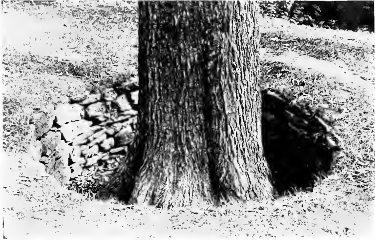
FIG. 29.—A “well” constructed about an elm-tree when grade was raised.
