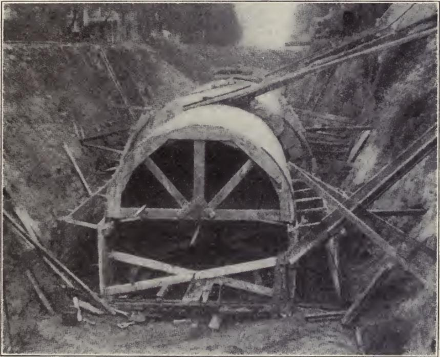
Fig. 42. Construction of Dry-Run Concrete Sewer, Waterloo; Iowa.
