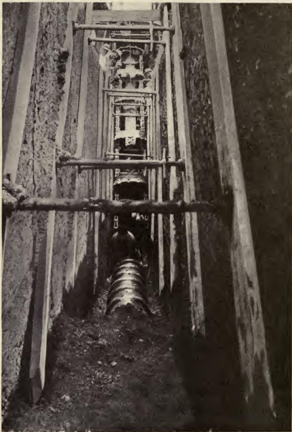
**AUSTIN TRENCHING MACHINE DIGGING TRENCH 18 FEET DEEP AND
