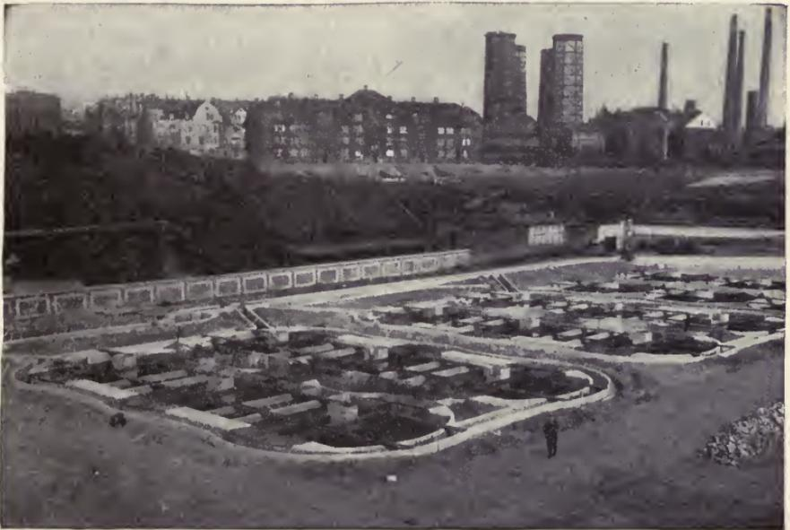
Fig. 53. Installation of Imhoff Tanks at Essen, North Germany
