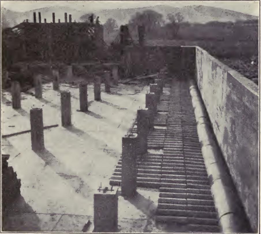
Fig. 64. Interior of Sprinkling Filter, Showing Underdrains Partly Laid
