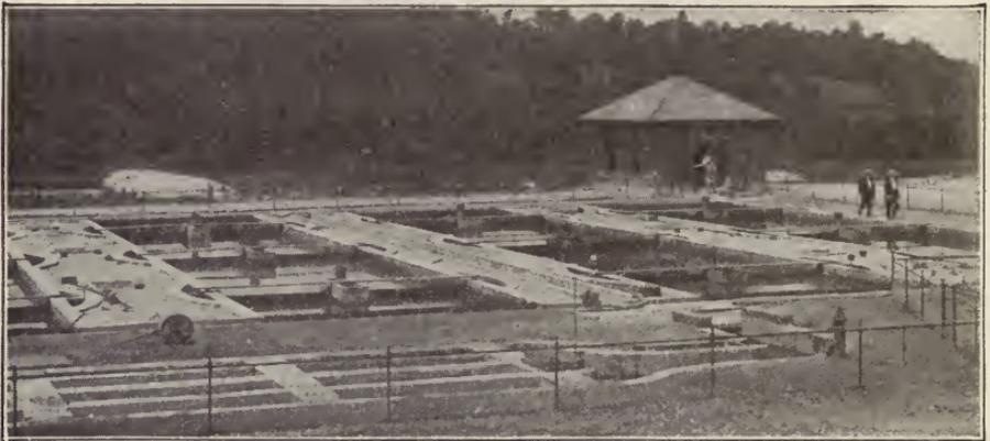
Fig. 51. Installation of Imhoff Tanks at Atlanta, Georgia
