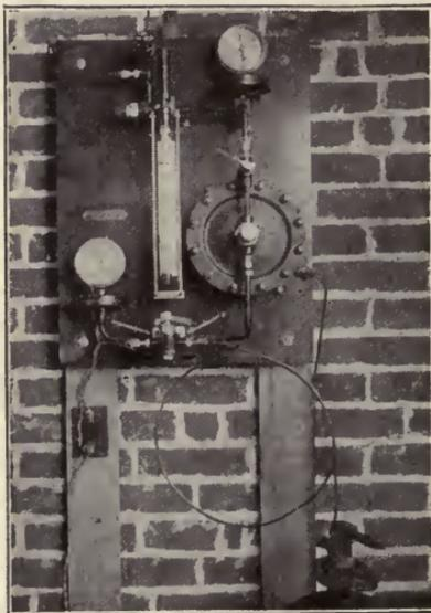
Fig. 68. Automatic Chlorinator
