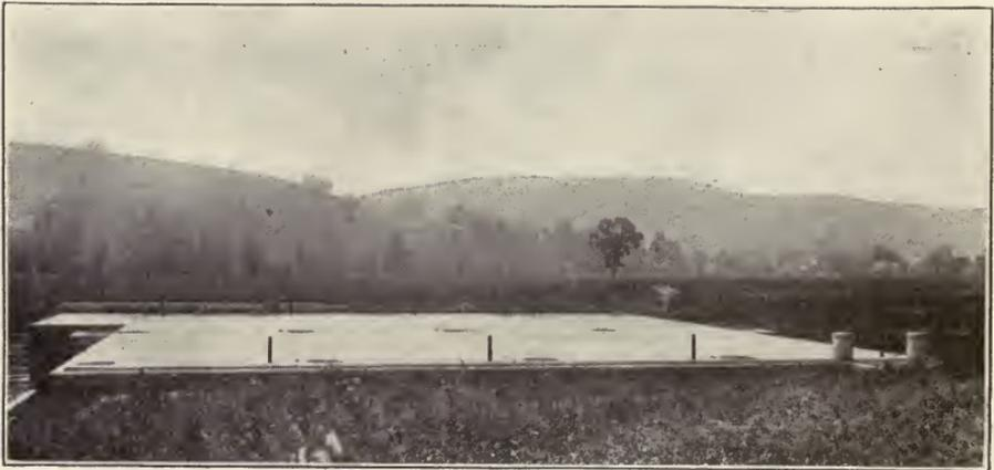
Fig. 48. Covered Settling Tanks of Polk Disposal Plant
