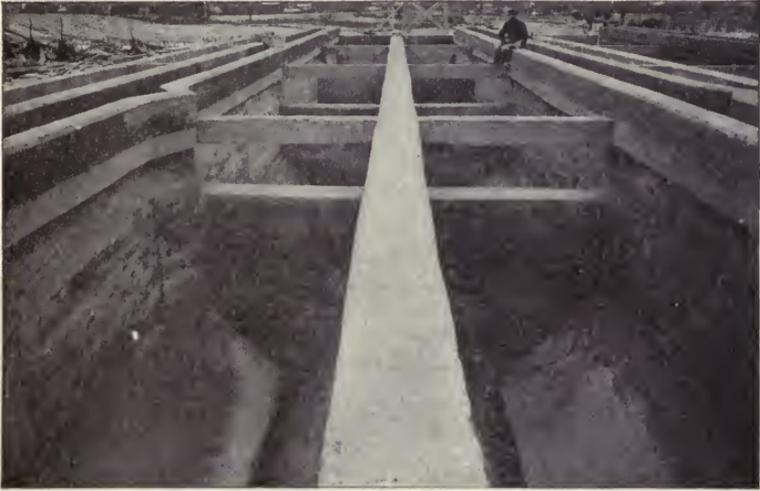
Fig. 52. Interior View of Imhoff Tanks at Batavia, New York
