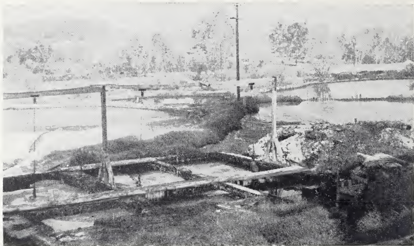
Figure 10.—Waste materials of a tannery are processed in lagoons from which the water is allowed to seep slowly into a small local stream, Luray, Va.
