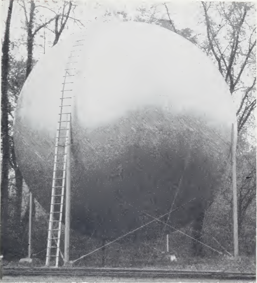
Figure 7.—The sewage disposal plant at Richmond, Ind., has a spherical storage tank for the combustible gases arising from the digestion chamber.
