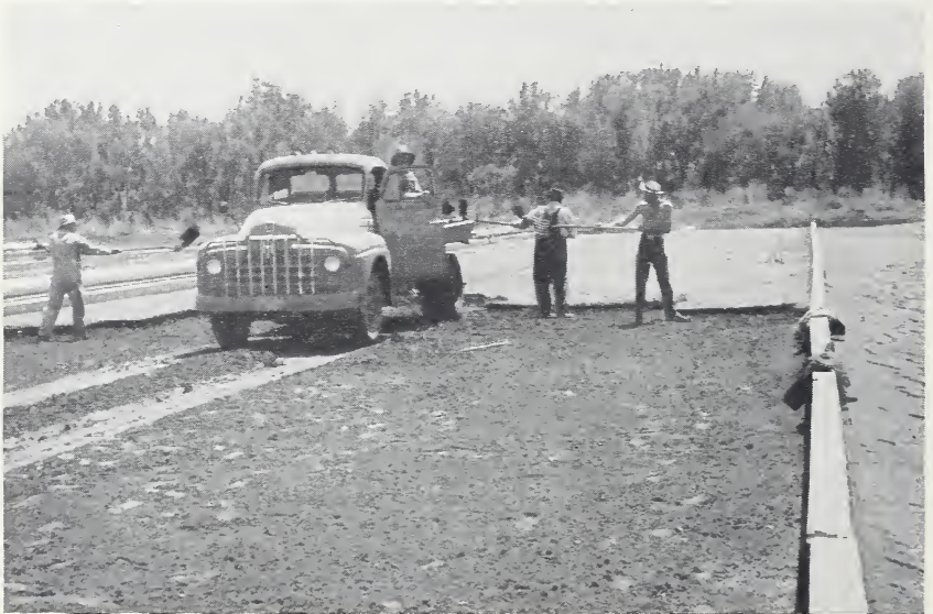
Figure 3.—Dried digested sewage sludge of the Des Moines, Iowa, plant is recovered for use as fertilizer.
