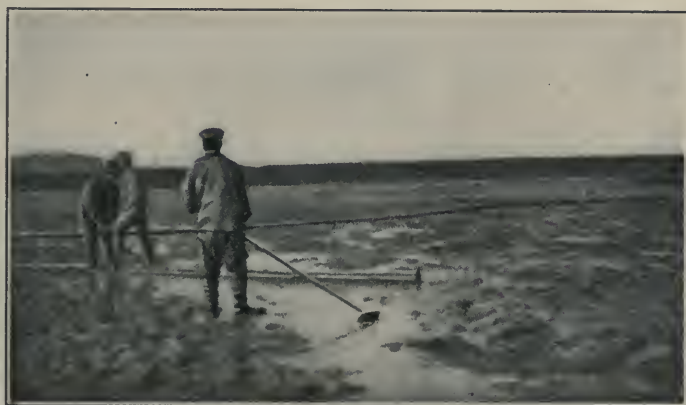
FIG. 29.—Sludge distribution pipes. (Mannheim.)
