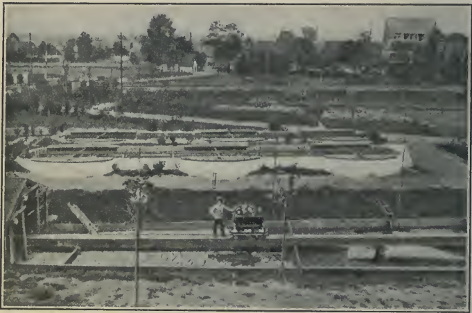
FIG. 21.—Sludge beds of the Recklinghausen Clarification Plant.
