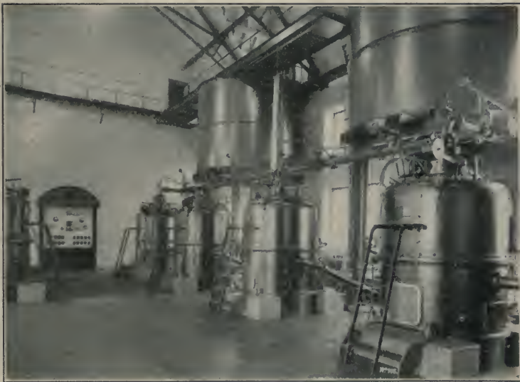
FIG. 41.—Centrifugal sludge-drying machine at Frankfort, Germany. (Courtesy of The Lathbury-d'Olier Co., Philadelphia.)
