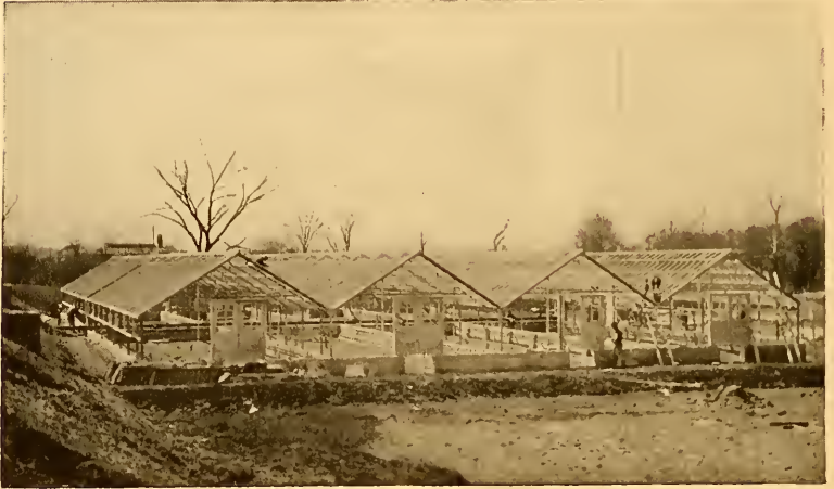
FIG. 125. Glass-covered Drying Beds at Alliance, Ohio.
