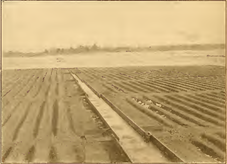
FIG. 69. Furrows and Sewage Distributors at Brockton, Mass. (courtesy of G. E. Bolling).
