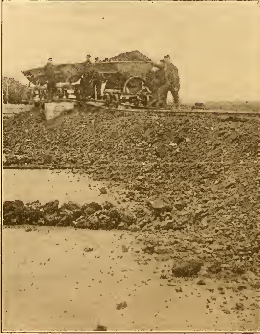
FIG. 82. Filling Contact Beds at Manchester.
