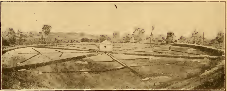
FIG. 83. General View of Contact Beds at Mansfield, Ohio.
