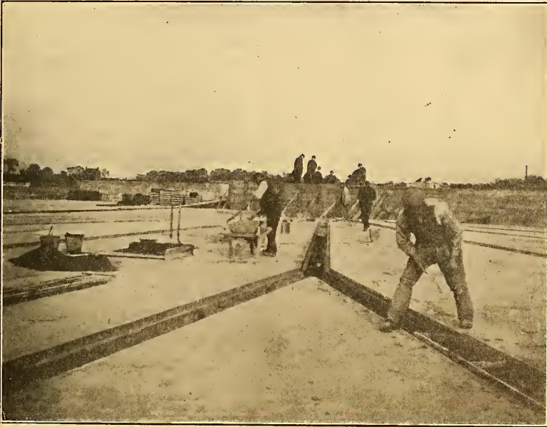
FIG. 76. Underdraining Contact Beds at Manchester.
