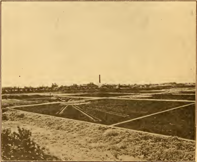
FIG. 78. Distribution of Sewage on Contact Beds at Manchester.
