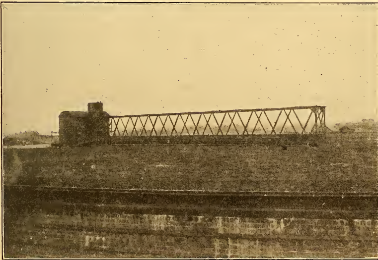
FIG. 96. Scott-Moncrieff's Revolving Distributor at Birmingham.
