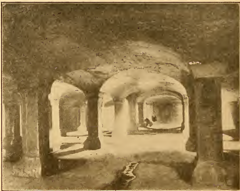
FIG. 45. View of Interior of Septic Tank at Saratoga, N. Y. (courtesy of F. A. Barbour).
