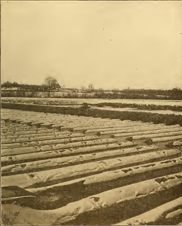
FIG. 73. Intermittent Filter Bed at Pawtucket, R. I., in Winter.
