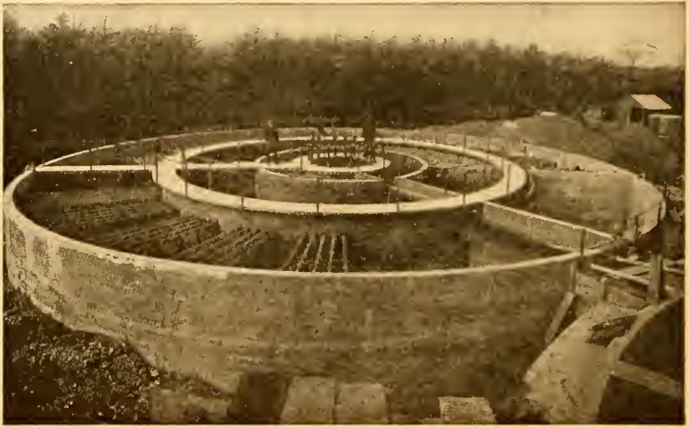
FIG. 52. Hydrolytic Sewage Treatment Tank, Luton, England (courtesy of Engineering News).
