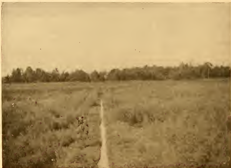
FIG. 62. Distributing Ditch, Moscow Sewage Farm.
