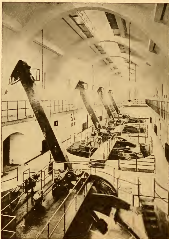
FIG. 23. Interior of Riensch-Wurl Screen House at Dresden (courtesy of The Sanitation Corporation).
