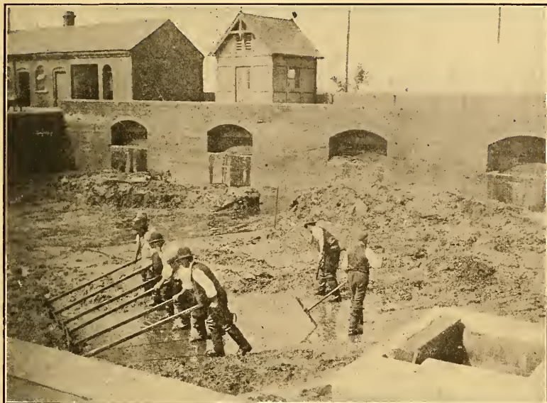
FIG. 34. Hand-propelled Squeegee used at Salford, England.
