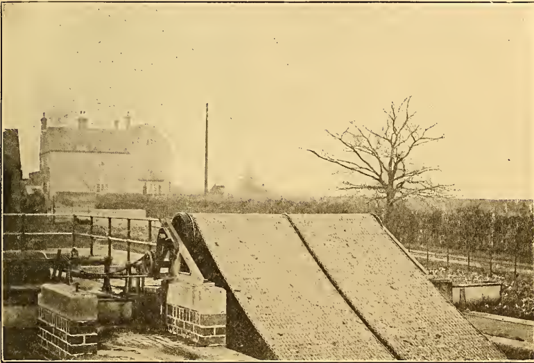
FIG. 16. Revolving Screen at Birmingham, England (courtesy of J. D. Watson).
