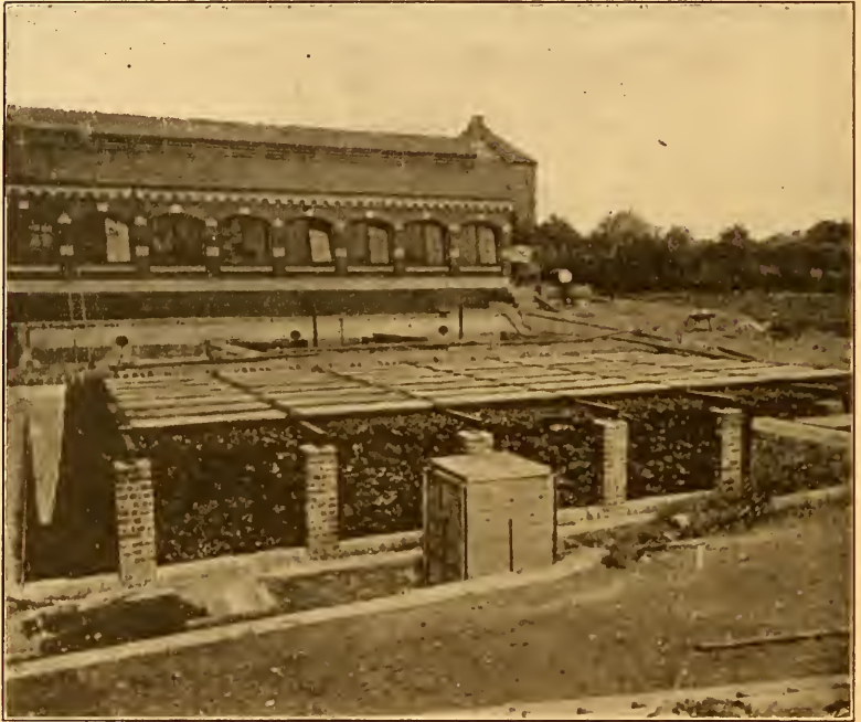
FIG. 90. View of Trickling Filter at Bristol (courtesy of F. Wallis Stoddart).
