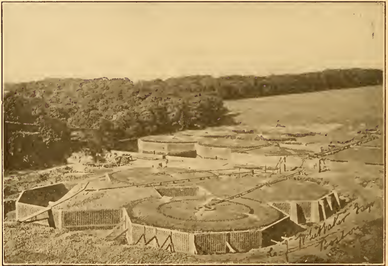
FIG. 92. Whittaker-Bryant Filter at Accrington (courtesy of Mr. Whittaker).
