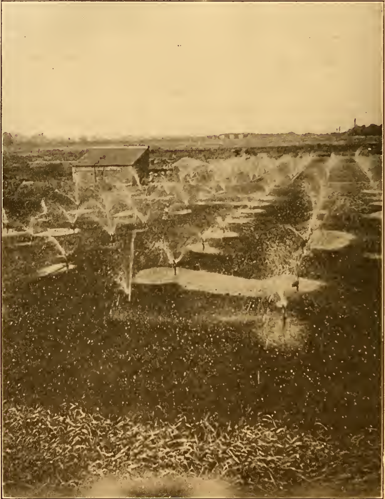
FIG. 107. View of Clogged and Pooling Trickling Filter.
