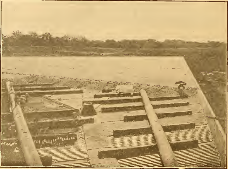
FIG. 113. View of Columbus Filters during Construction (courtesy of J. H. Gregory).
