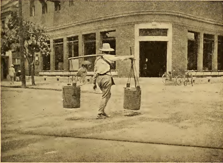
FIG. 1. Removal of Night-soil, Tokyo.
