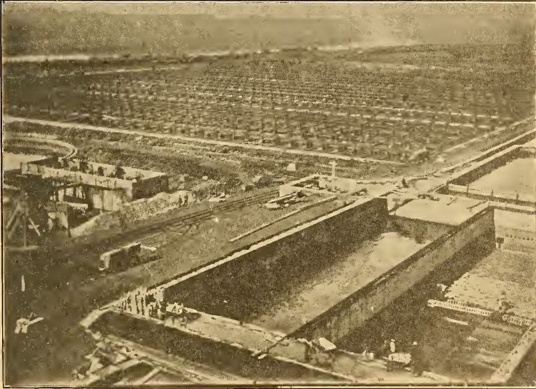
FIG. 110. General View of Salford Beds during Construction.
