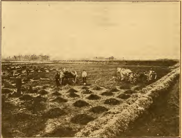
FIG. 123. Scraping Intermittent Filtration Beds in Spring, Worcester Sewage Works.
