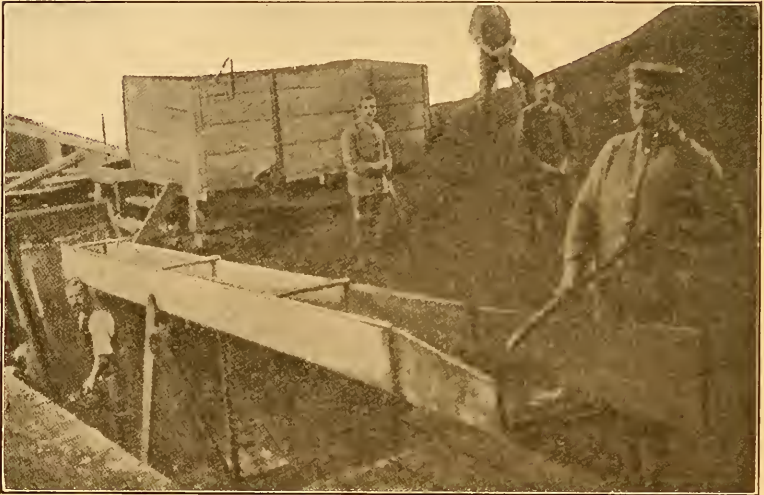
FIG. 81. Washing Contact Material by Hand at Hamburg (copied by permission from Dunbar, 1908).
