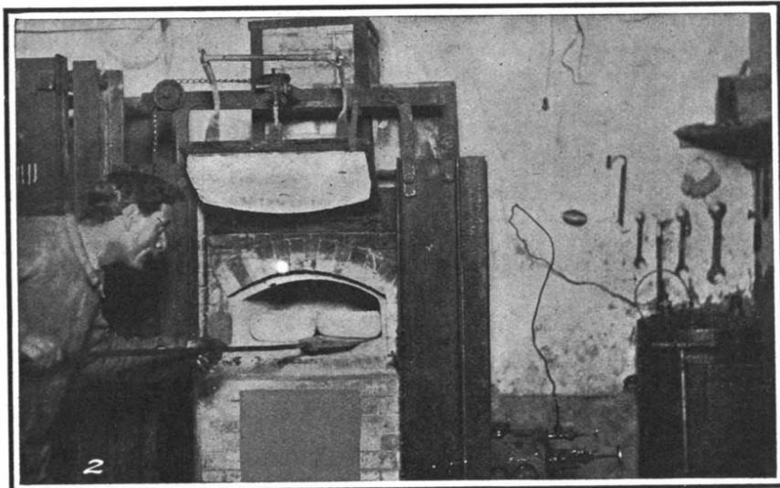
Thrusting the crucible into the furnace.
