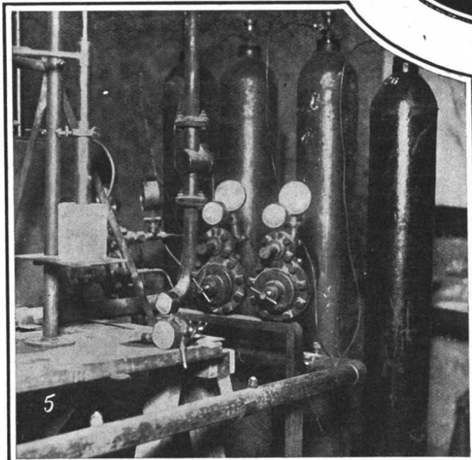
Oxygen tubes feeding a row of blowpipes.
