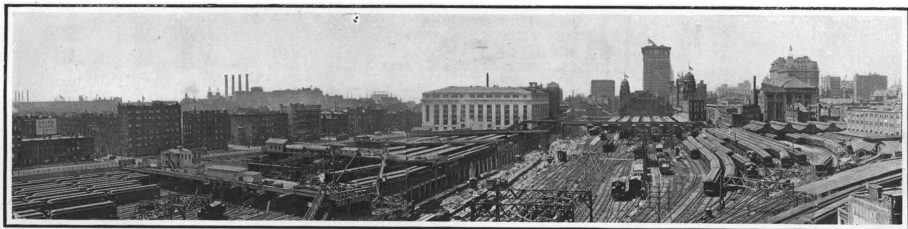
The completed portion of new yard.
