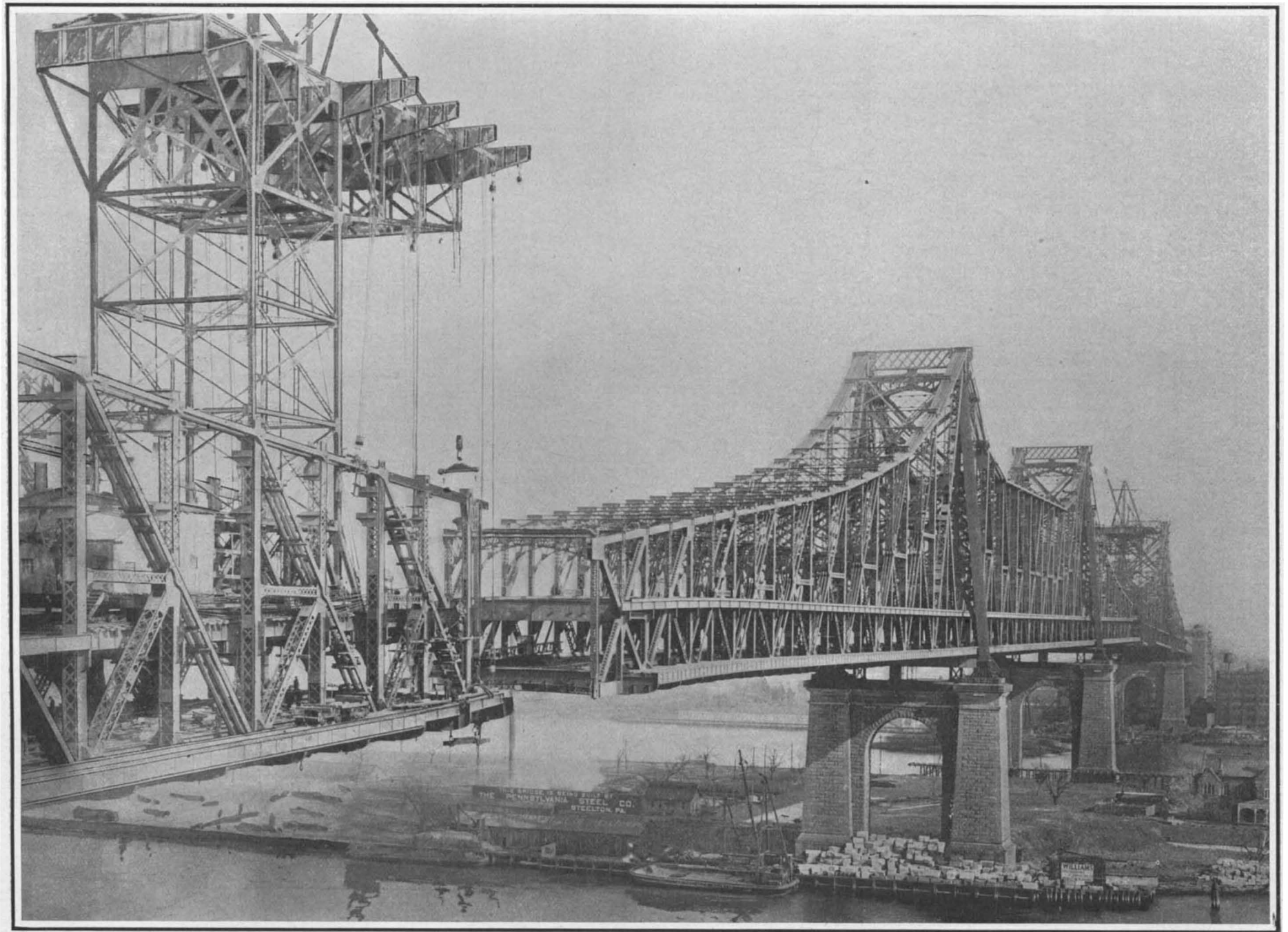
Total Length of Bridge, Including Approaches, 7,408 Feet. Total Length of Cantilevers, 3,727 Feet. Total Weight of Cantilevers, 52,000 Tons. Bridge Has Two Floors, Accommodating Eight Tracks; a 36-Foot Driveway, and Two 13-Foot Sidewalks for Pedestrians. The Strongest and Heaviest Bridge in the World, Able to Carry 8 Tons to Each Foot of Its Length.
