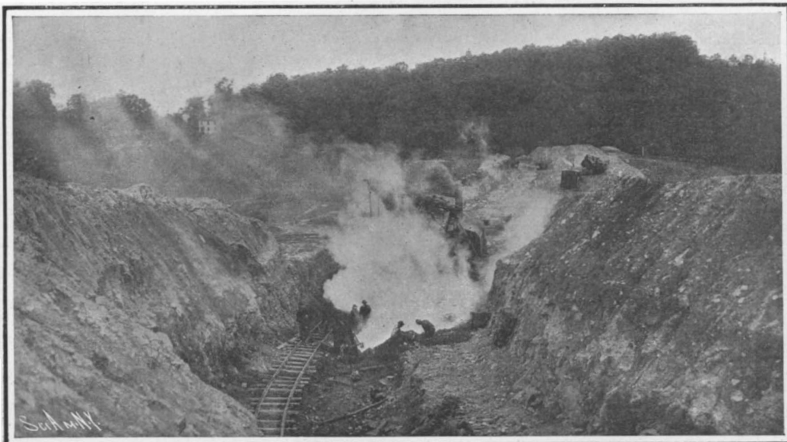
Excavation of Trench Preparatory to Building the 17½-Foot Concrete Aqueduct. The Aqueduct Will be Constructed Upon a Carefully-Leveled Foundation and Covered in with Earth Rolled Down in Layers.
