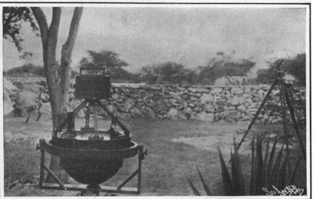
Ship Horizontal Force Instrument Mounted on Tripod for Shore Observations at the Honolulu Magnetic Observatory, September, 1907.
