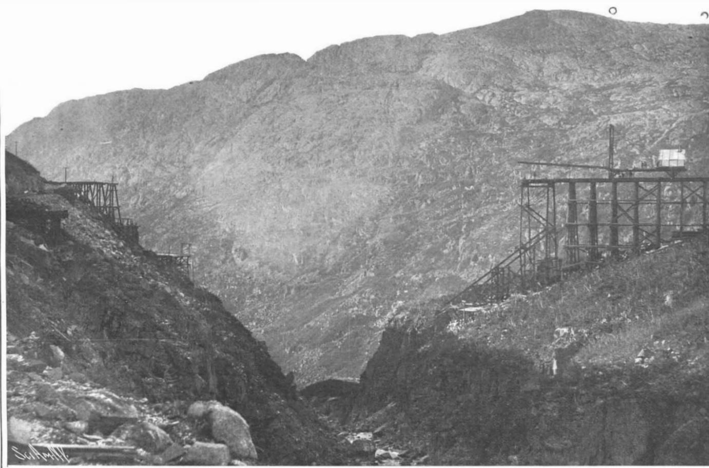
The Steel Cantilever Bridge Spanning the Canyon, in Process of Construction.
