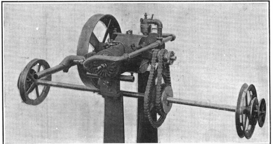
**ENGINE AND TRANSMISSION OF THE HOLSMAN CARRIAGE-TYPE AUTOMOBILE.**
