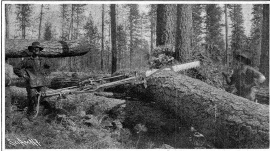
The Compressed-Air Logging Saw in Operation.
