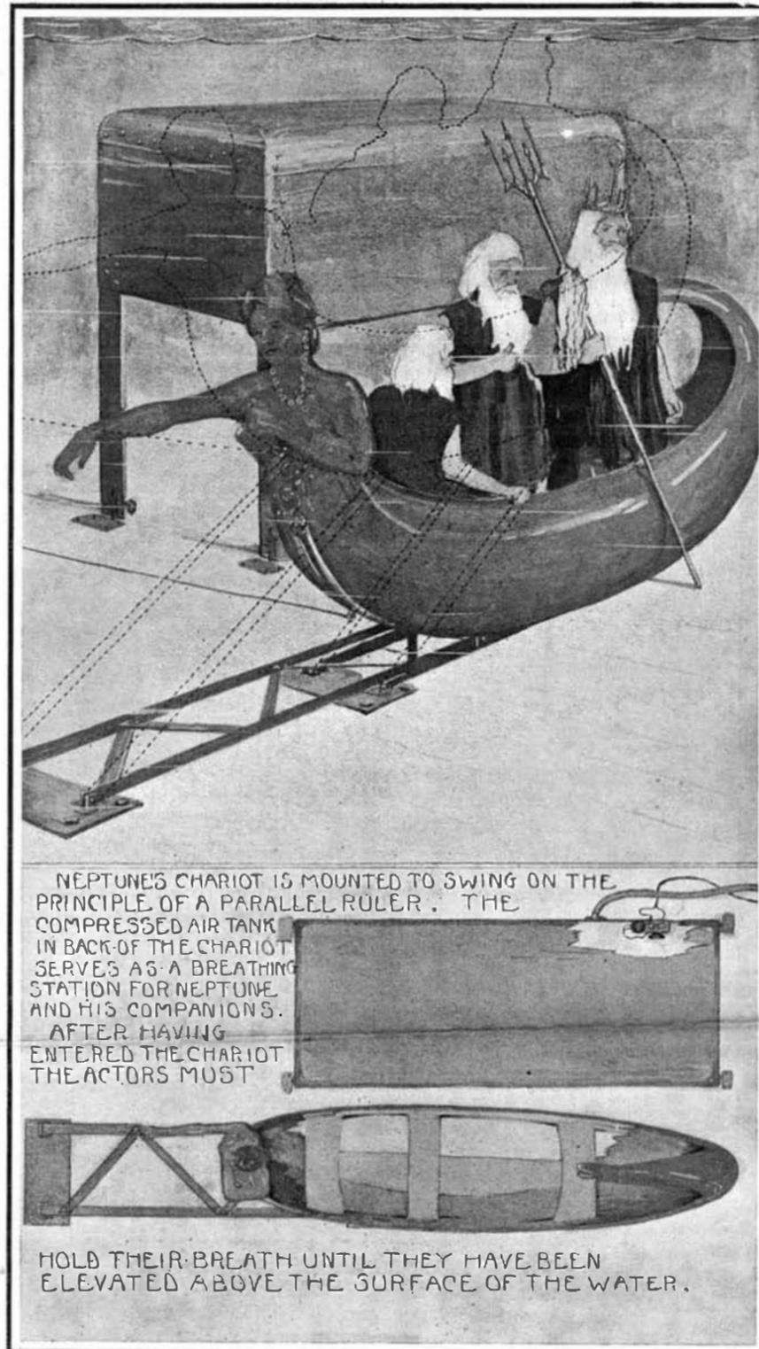
The Elevating Device at Rest Just Prior to Raising.
