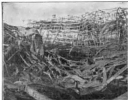
Effect of fire on unprotected steel—so-called "fire-proof" construction. Name and location of above building sent on request.
