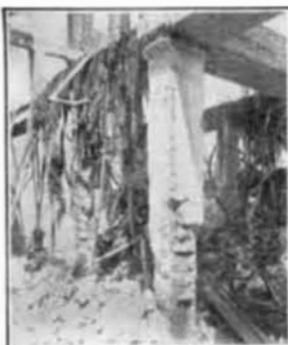
Effect of fire on reinforced concrete structure. A so-called "fire-proof" building. Name and location of above building sent on request.
