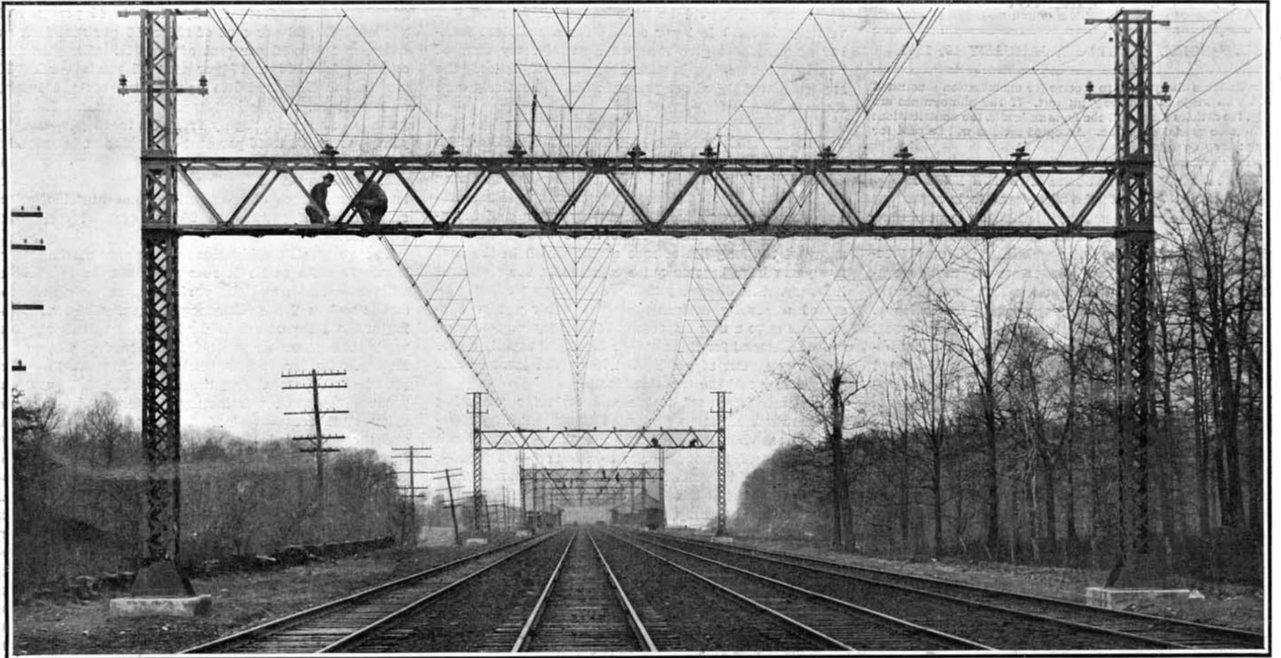
Each catenary consists of two  $\frac{1}{4}$ -inch steel cables carried on insulators on the top of the trusses. The copper trolley wire is suspended from the cables and held in level and alignment by triangles made of  $\frac{3}{8}$ -inch pipe.
