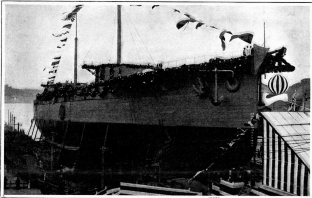
**Length, 482 feet. Beam, 83½ feet. Displacement, 19,200 tons. Horse-power, 18,000. Speed, 20 knots. Armor: Belt, 9½ inches. Armament: Four 45-caliber 12-inch; twelve 45-caliber 10-inch; twelve 50-caliber 4.7-inch. Torpedo tubes, 5.**
