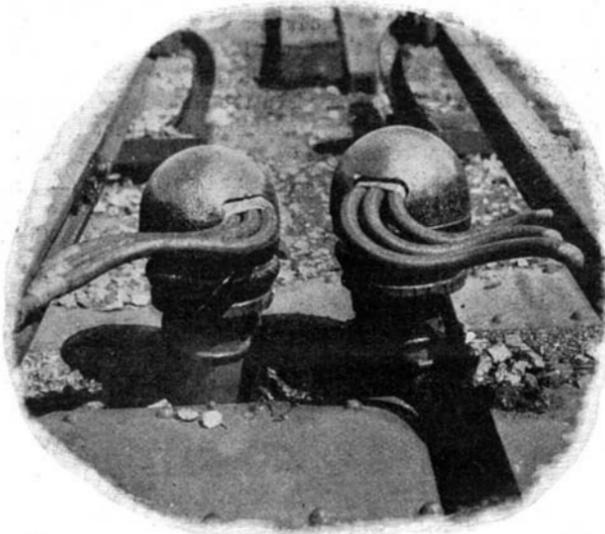
Third-Rail Jumper Connections Used at Cross-Overs.
