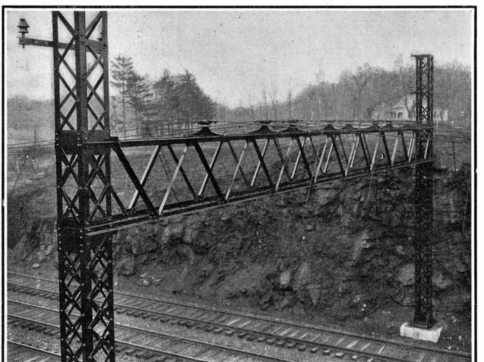
Near View of Steel Posts and Truss, Showing Method of Attaching Catenaries.
