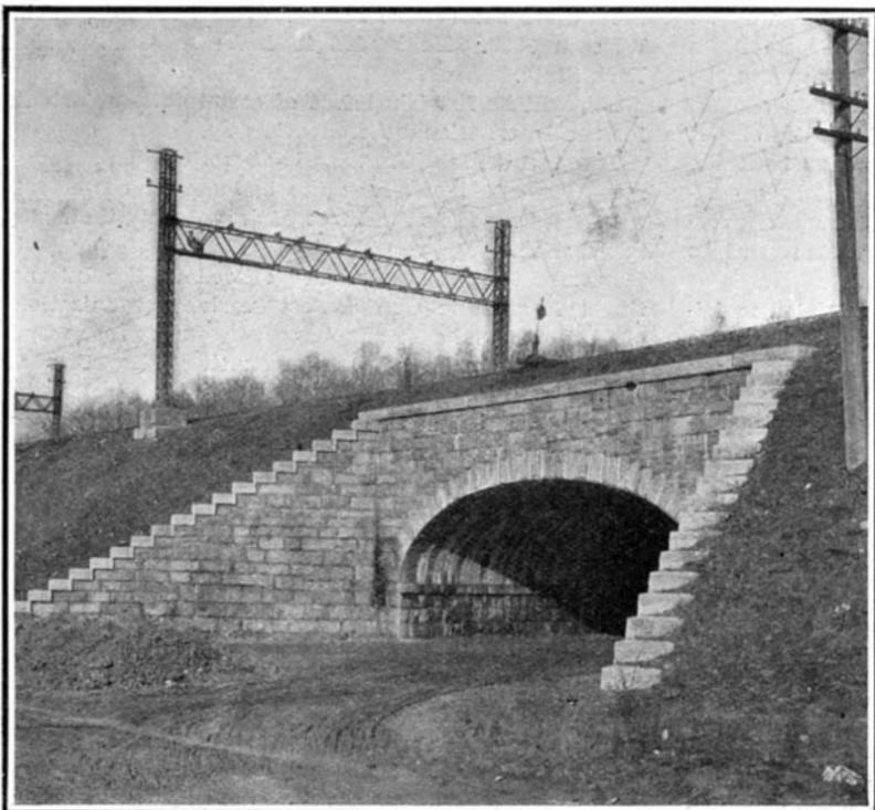
A Sketch of the New Haven Trolley Lines, Showing the Method of Stiffening by Triangles.
