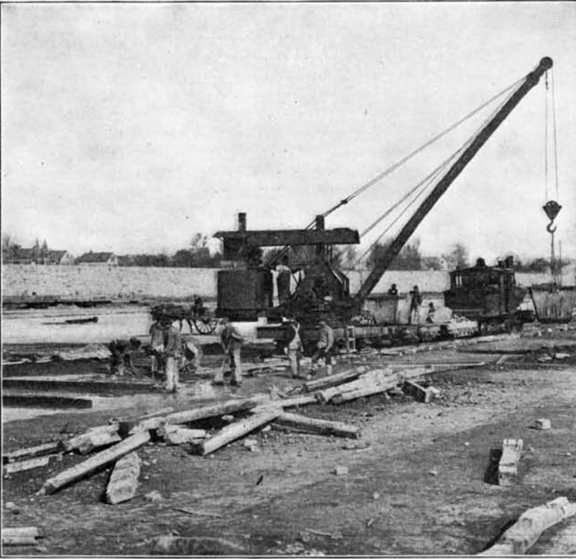
Laying the Concrete Floor in the Reservoir.
