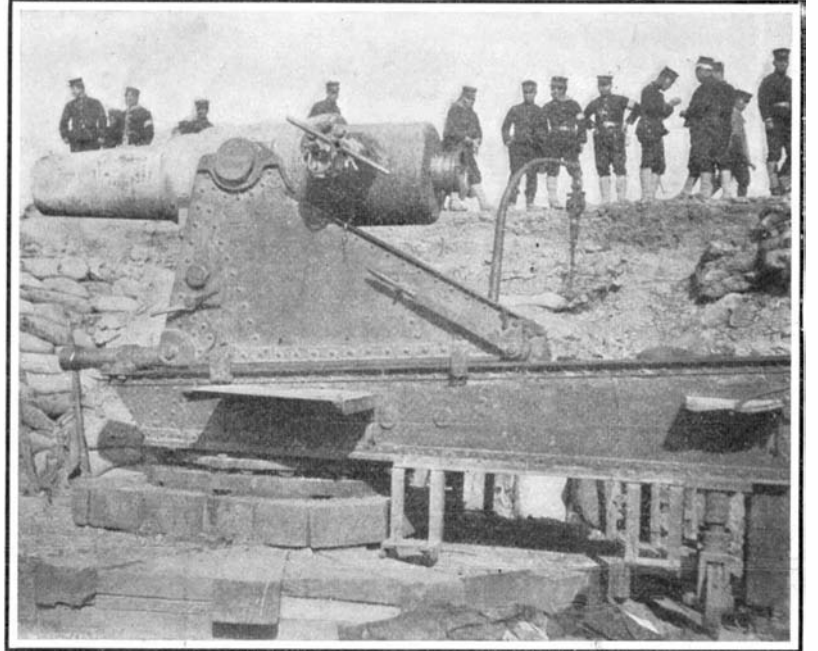
Heavy Mortar on an Improvised Foundation.
