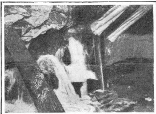
Springs Gushing from Tunnel Walls.
