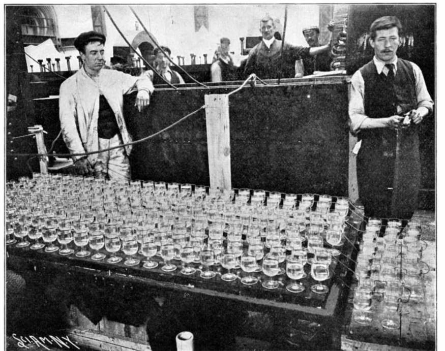
Testing a Cable. A 20,000-Volt Current is Passing Through the Goblets.
