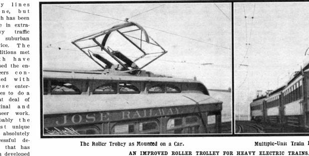
gears at the bottom cause the side frames to move in unison, while the gears at the top keep the guards always in a vertical position, as shown. The roller is carried at the top on a shaft, the ends of which are fastened rigidly in a casting to which the guards are secured and on which pivot the segmental gears. The roller is made of 24 inches of 5-inch non-arcing metal
