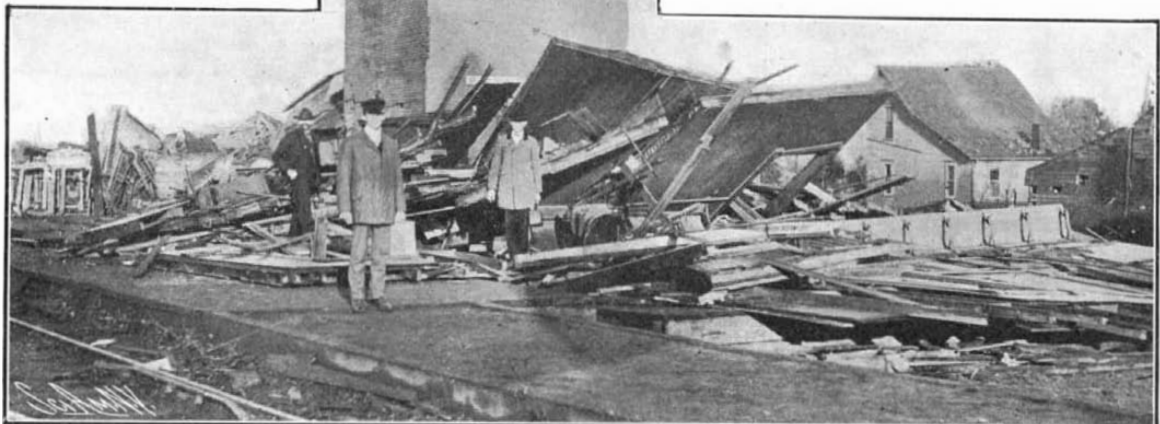
Scene at the Railway Station, Showing the Ruins of the Depot and What is Left of the Grain Elevator.
