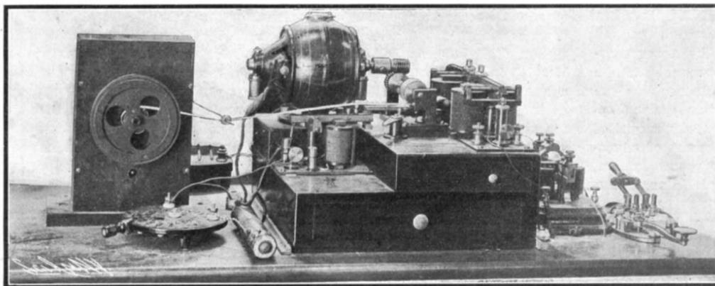
**Machine for Perforating the Transmitting Tape.**
