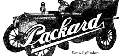
Actual 22 horsepower, with only 85 lbs. loaded weight to each horsepower. Speed range of 4 to 40 miles per hour. Anti-friction ball bearing axles, direct drive, mechanical valves for intake and exhaust. Winner of highest prizes for BOTH speed and endurance wherever entered.
