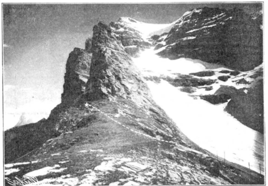
The Rothstock Station (Located Back of the Star). Altitude 8,270 Feet. The Dotted Line Shows the Course of the Road Through the Rock.
