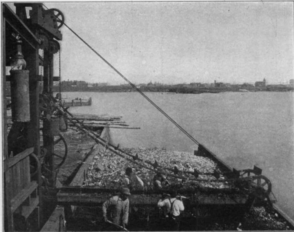
Automatic Conveyor for Unloading Garbage.
