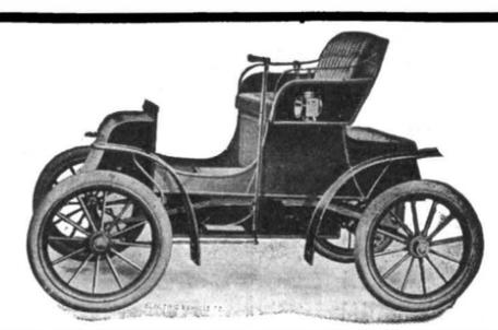
Fastest, handsomest and most convenient Electric Runabout on the market. Five speeds up to 15 miles per hour. Underlump battery and motor, leaving body space entirely free for luggage.
