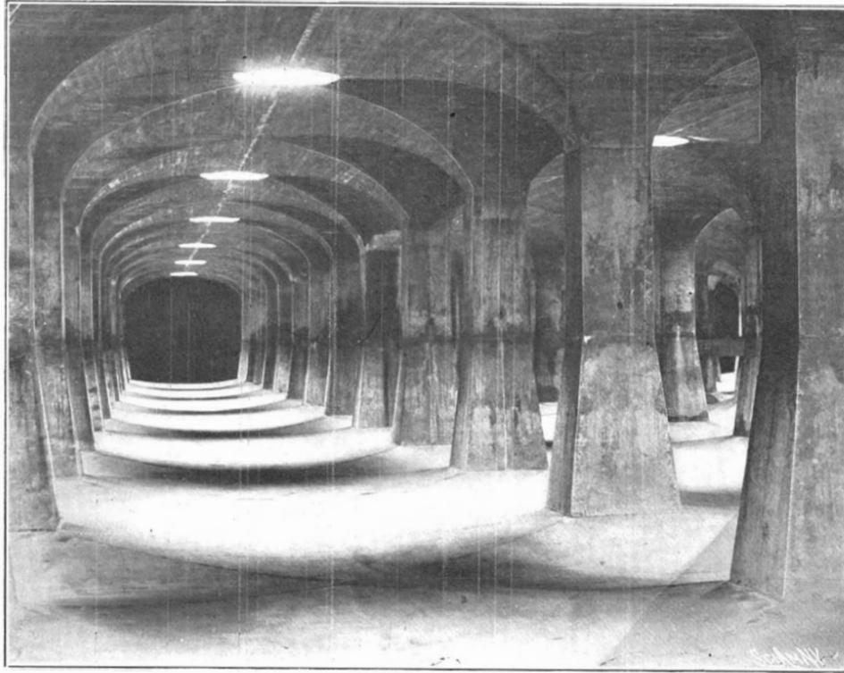
Perspective View of One of the Compartments of Filter Bed.
