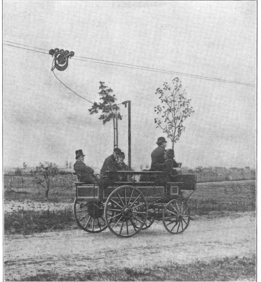
Electrical Wagon Operated by Auto-Motor Trolley.
