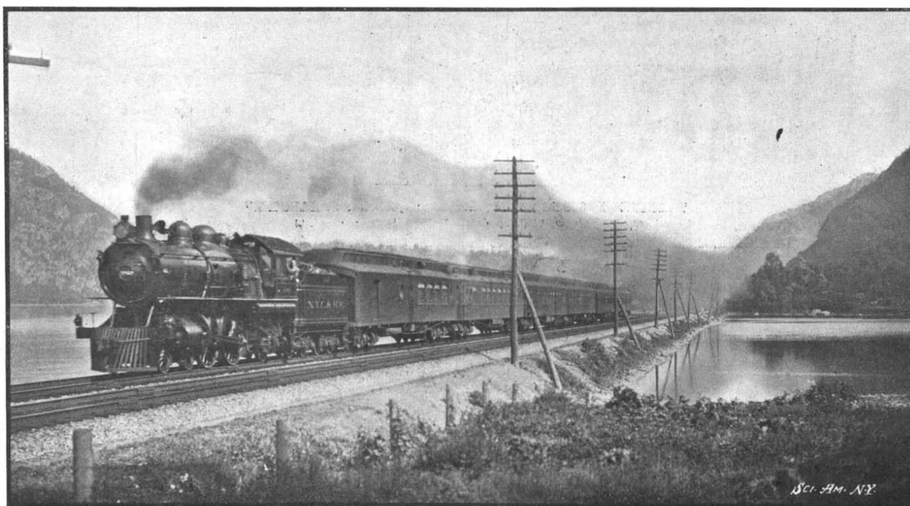
Albany to Spurtin Duyvil, 131.7 miles, was run in 131 minutes. Excluding the time lost in eight slowdowns, the average running speed was 68 miles per hour; weight of train, 352 $\frac{1}{2}$  tons; of engine, 144 tons.
