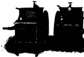
Fire protection for R.R. wrecks, carried on wreck trains, two 45 gallon Chemical Fire Engines on wheels, easily handled. Four men can lift over obstructions. Space required 5 feet wide, 6 feet long and 4 feet high. Will throw a stream of chemicals 40 to 50 feet for hours. Equal in fire extinguishing capacity to 3 1/2-in. streams of water.
