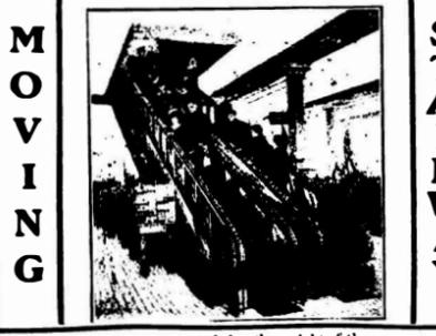
The Elevators are so constructed that the weight of the passengers descending assists in raising the ascending passengers; consequently the cost to operate them is small. Booklet free. **The Reno Inclined Elevator Co., 551 W. 85th Street, New York.**
