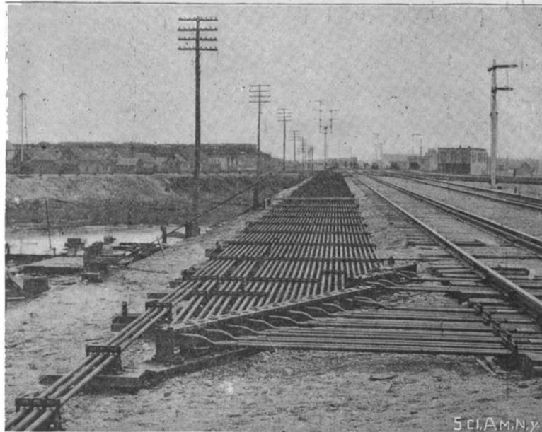
Fig. 6.—Connections from Cabin to Switches and Signals.
