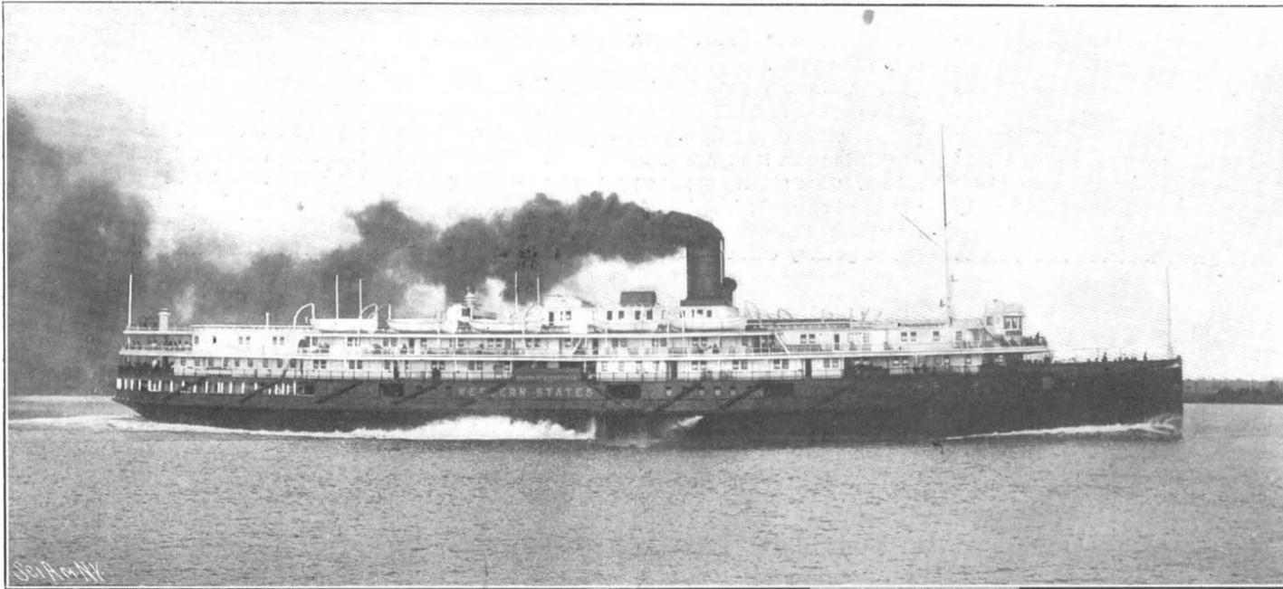
Length over all, 386 feet; breadth, 44 feet; depth, 26 feet; tonnage, 5,000; horse power, 8,000; draught, 16 feet 8 inches; speed, 22 miles an hour.
